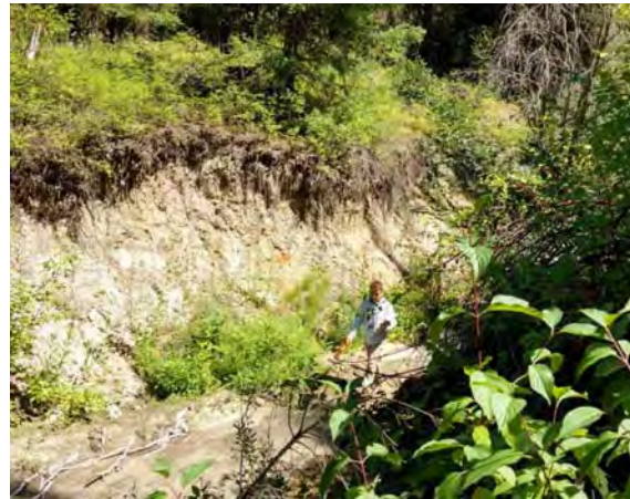
Stream Channel Erosion
