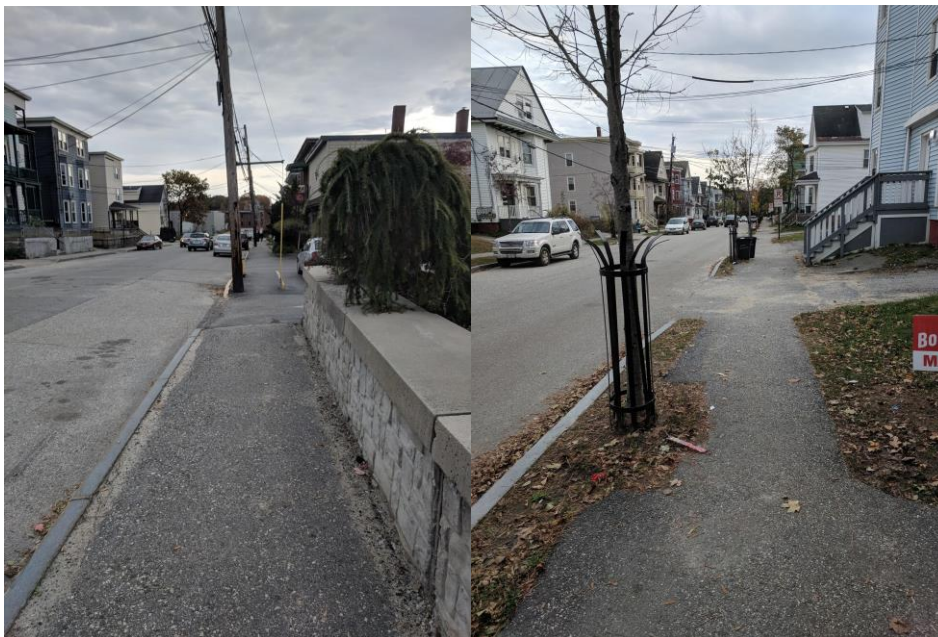
Figure 7: Comparison between our sidewalk smoothness evaluations and the focus group's. On the left (Park Street between Birch and Maple), we evaluated the sidewalk as a 4 and the focus group (on average) evaluated it as a 2.1. On the right (Horton Street between Walnut and Birch), the focus group evaluated it as a 2.8 (average) and we evaluated it as a 1.
