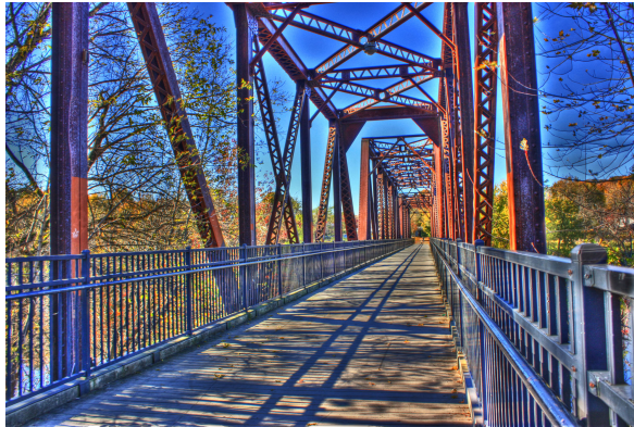
Railroad Bridge, connecting Lewiston & Auburn
