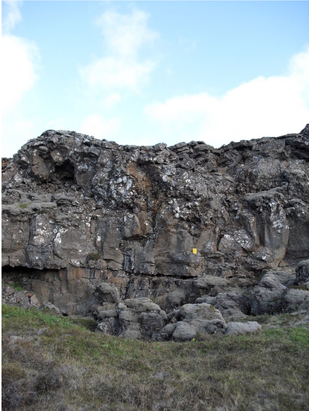
Figure 3.7 Picture of fault P, representing a typical vertical scarp seen in the field. Field notebook for scale.
