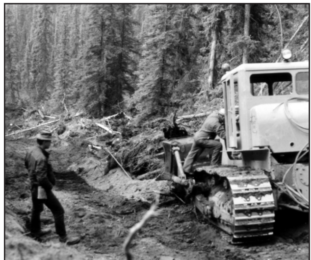
Bill Meadows (ANC-66) checking out disabled dozer. (Courtesy Major Boddicker)
