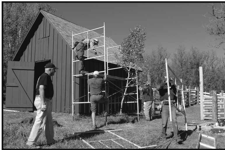
Building Restoration & New Fence
