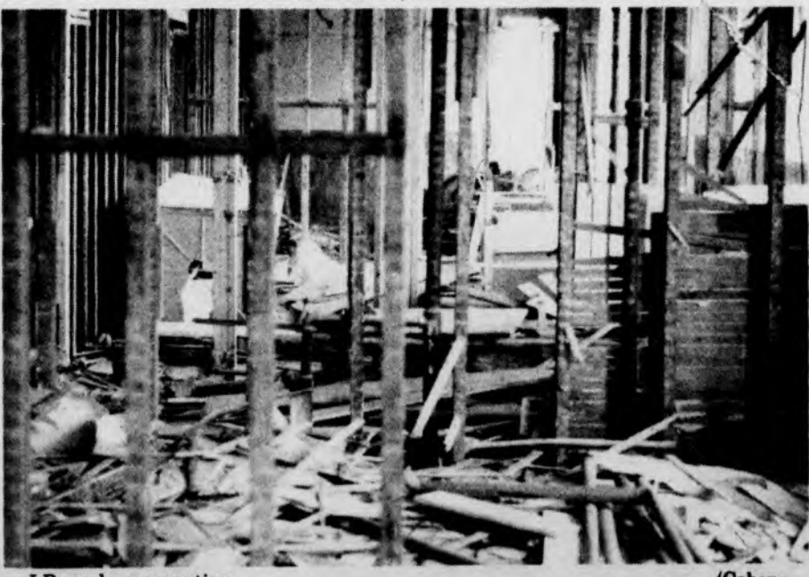
J.B. under renovation
