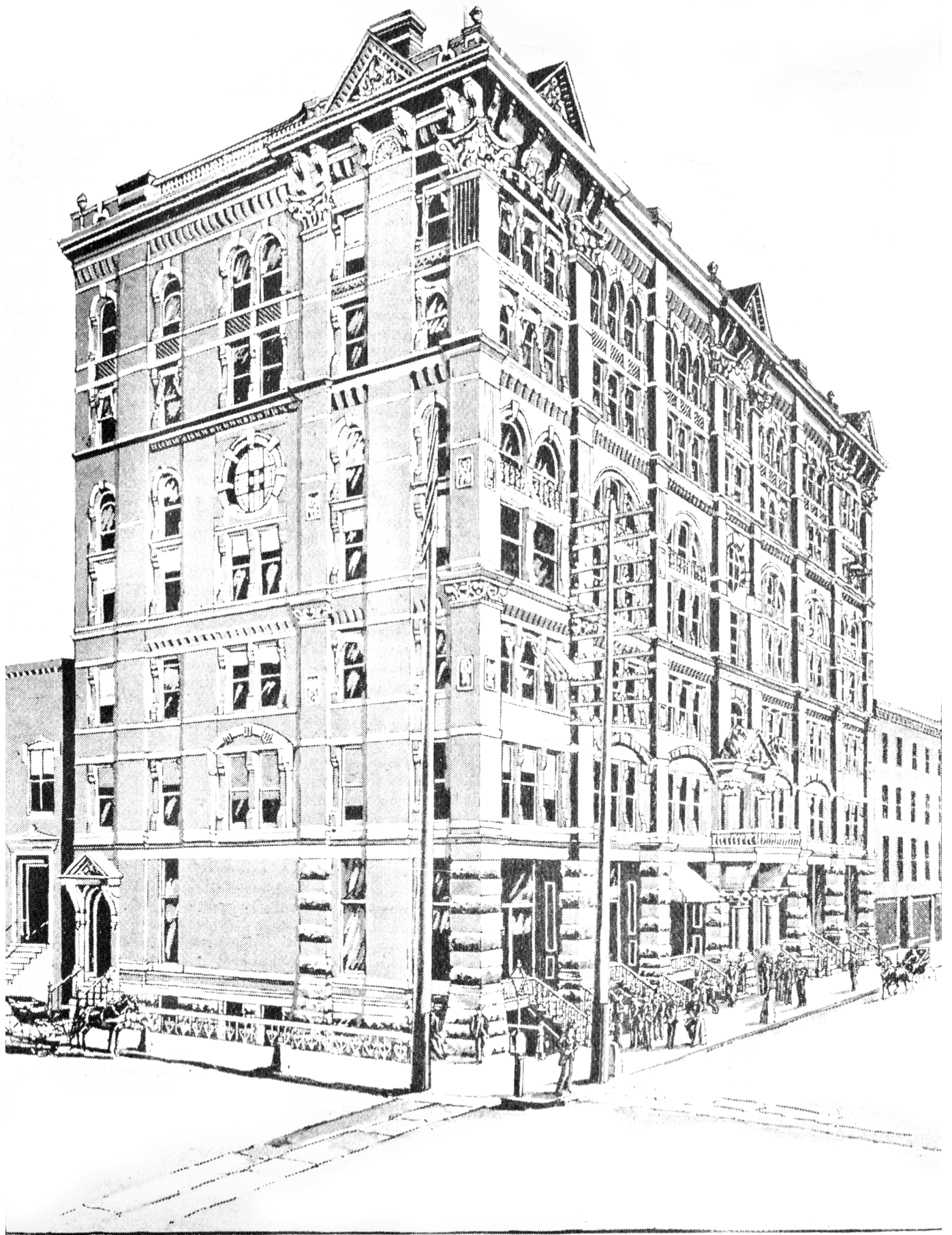
MERCHANTS' EXCHANGE; BOARD OF TRADE BUILDING.
