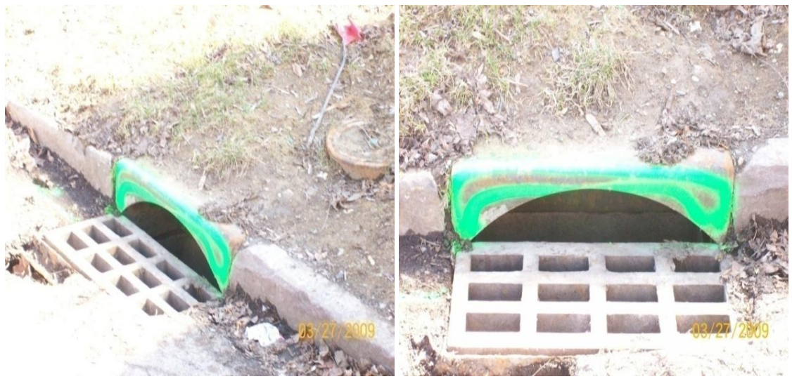
Figure 15.Photo# 15; Figure 16. Photo #16: Spray Painted Sewer Opening
