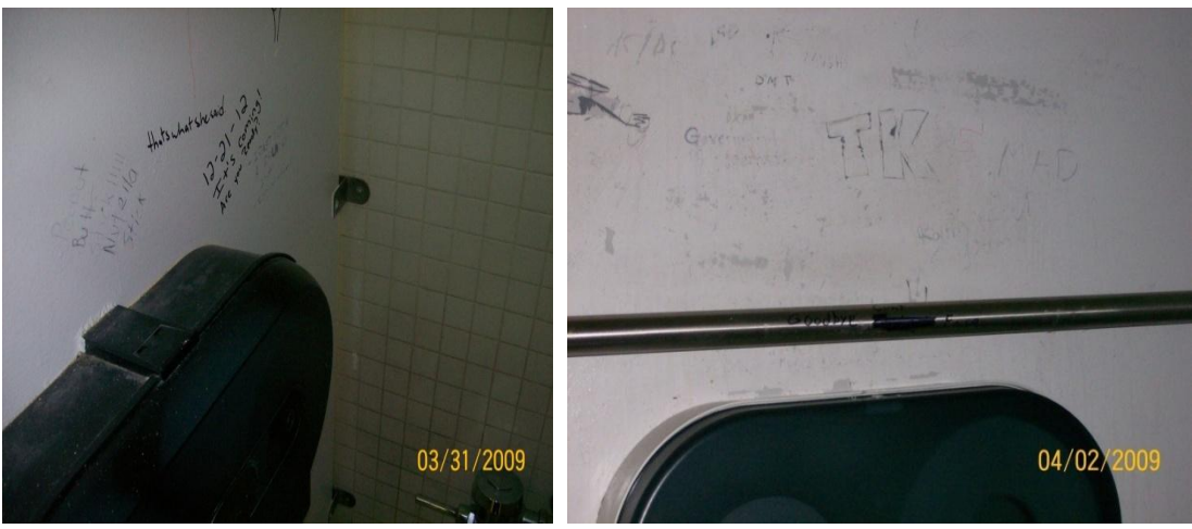
Figure 19.Photo #19; Figure 20.Photo #20: Writings in the Stalls of Public Bathrooms
