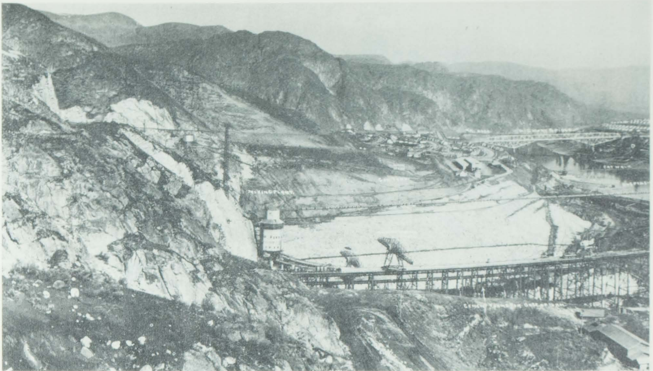
PANORAMIC VIEW OF GRAND COULEE DAM CONSTRUCTION. UPPER PLATE SHOWS WEST SIDE WITH ENGINEERS TOWN IN BACKGROUND. LOWER PLATE SHOWS EAST SIDE CONSTRUCTION WITH MASON CITY IN BACKGROUND.
