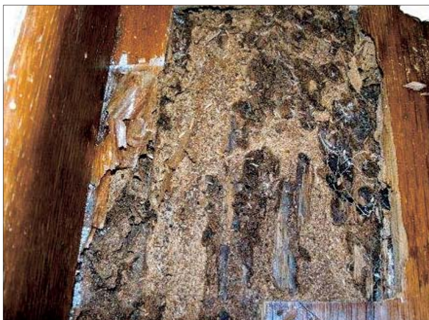
Fig. I – Strips of the parquet of the gym monitored in the study area, showing the typical signs of attack by subterranean termite. The wood appears lined with termite droppings, that being rich in moisture tend to clot and stick to the point where they are released. The droppings, mixed with soil and saliva, are used to construct the cells and galleries occupying the space freed by the wood consumption, forming the so-called “replacement wood”.
