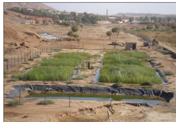
Figure 5 - Oasis of Brézina (Algeria) – view of the constructed wetlands in October (2013).
