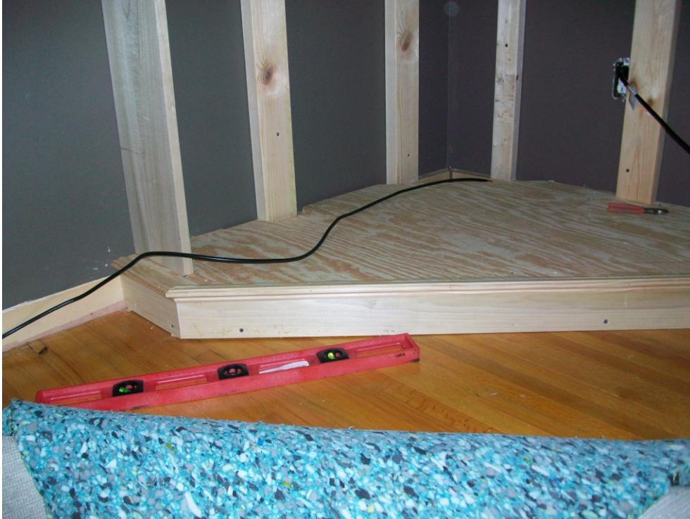
Figure B 13. The second side panel was attached.
