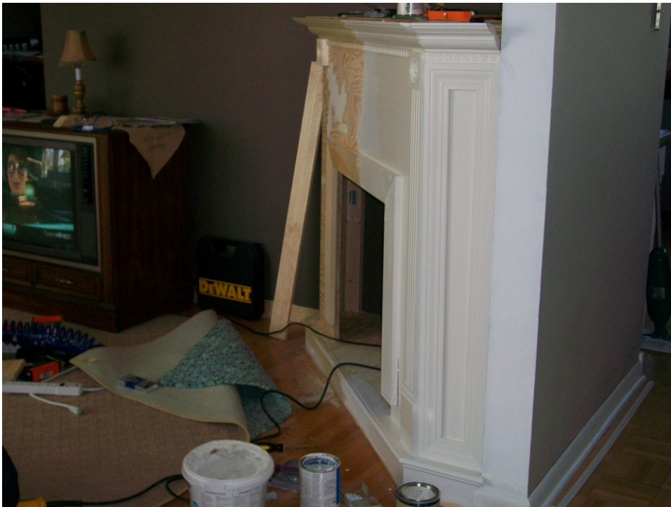
Figure B 22. The wood needed to be primed before painted.
