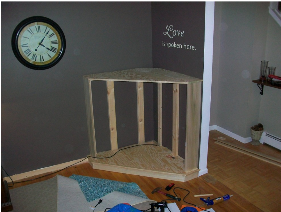
Figure B 14. I cut the top piece of 1" plywood. I waited to permanently attach it until after the front panel was secure.
