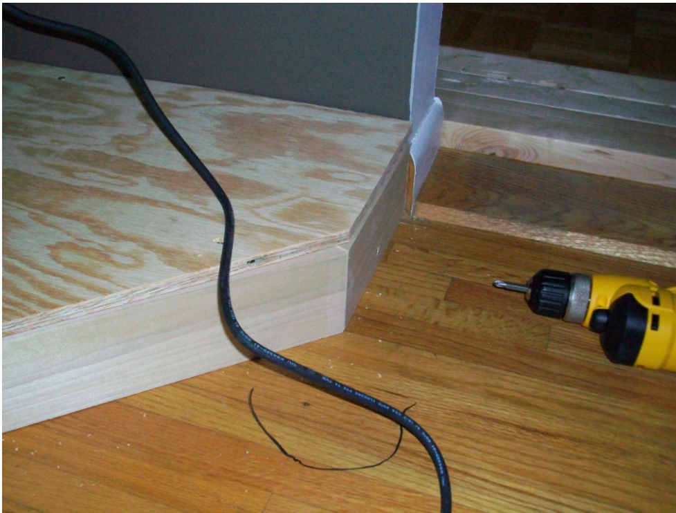
Figure B 6. This is a close up view of hearth's edge before the molding is added.
