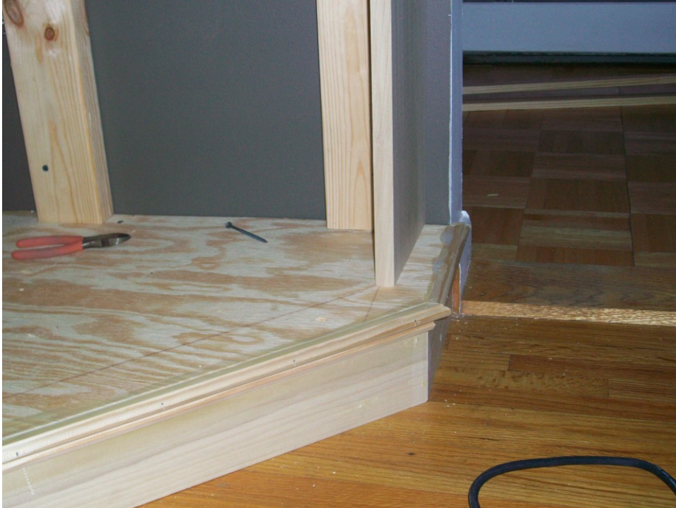
Figure B 7. This is a close up view of hearth after the molding is attached.
