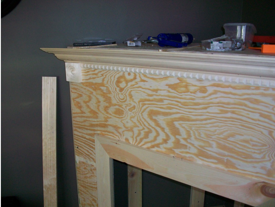
Figure B 19. I began attaching dentil molding and decorative pieces to give my project visual interest.
