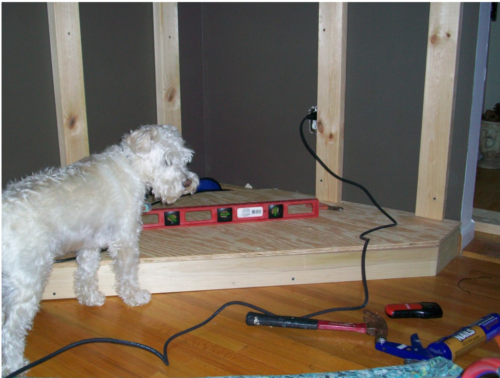
Figure B 8. This is Reggie, checking out my work. I was constantly checking that the structure was level.
