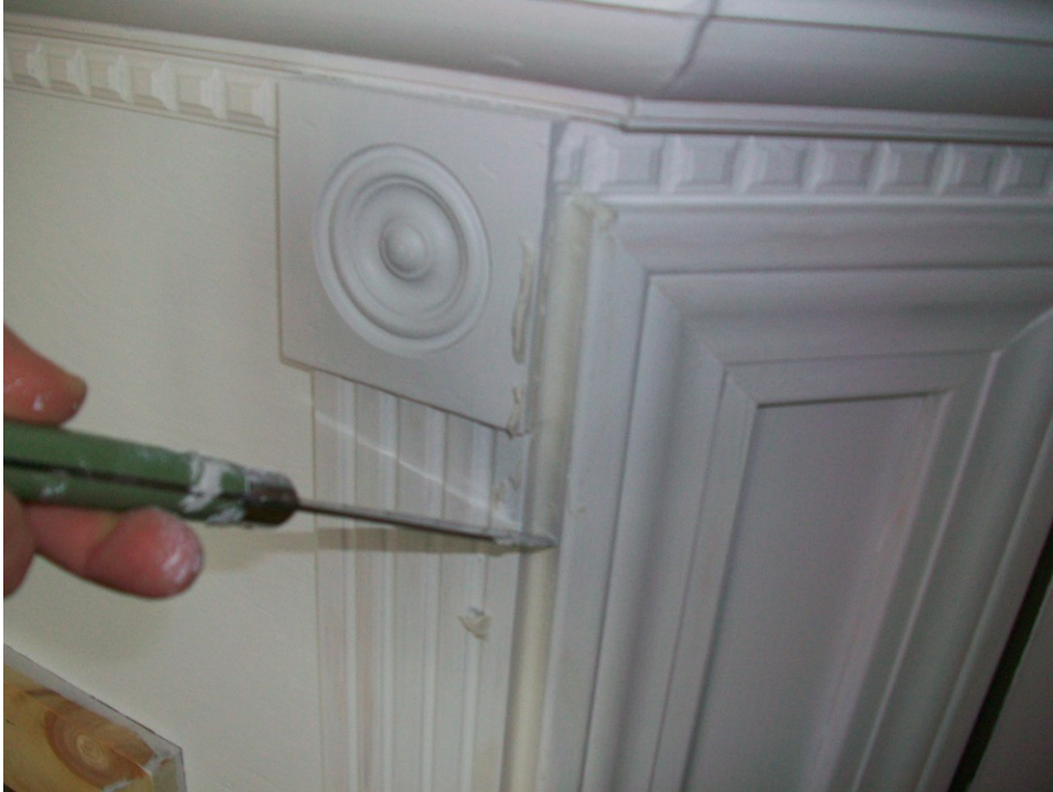
Figure B 23. I used joint compound to fill in any gaps.
