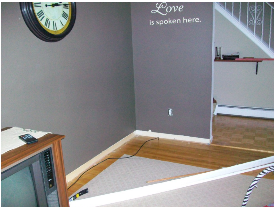
Figure B 2. The baseboard and shoe molding was removed.
