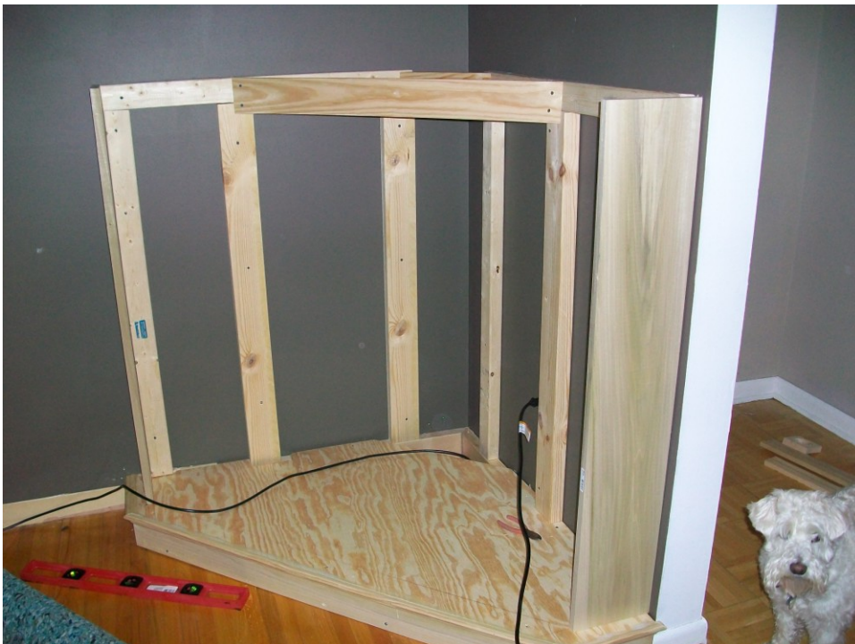
Figure B 12. This is the poplar side panel attached to the 2x4 support beam.
