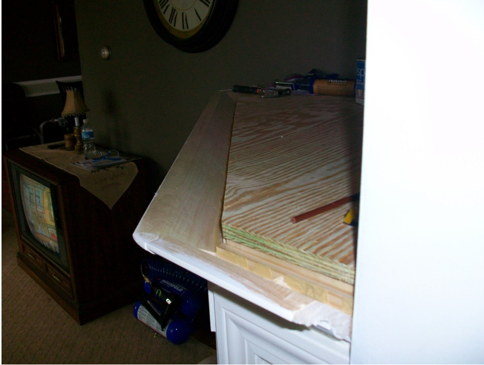
Figure B 21. This is another view of the hollow mantle before the thin birch plywood was attached on the surface.
