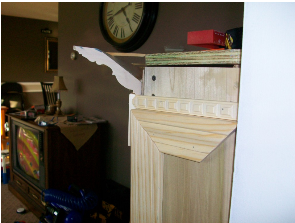
Figure B 18. The mantle is hollow and that is visible from this angle.
