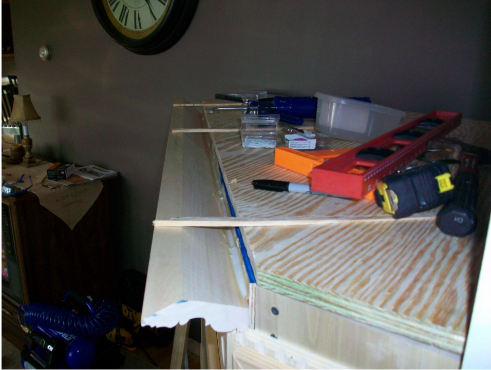
Figure B 17. Once the front piece was secure, I began to add the crown molding that will serve as the mantle.
