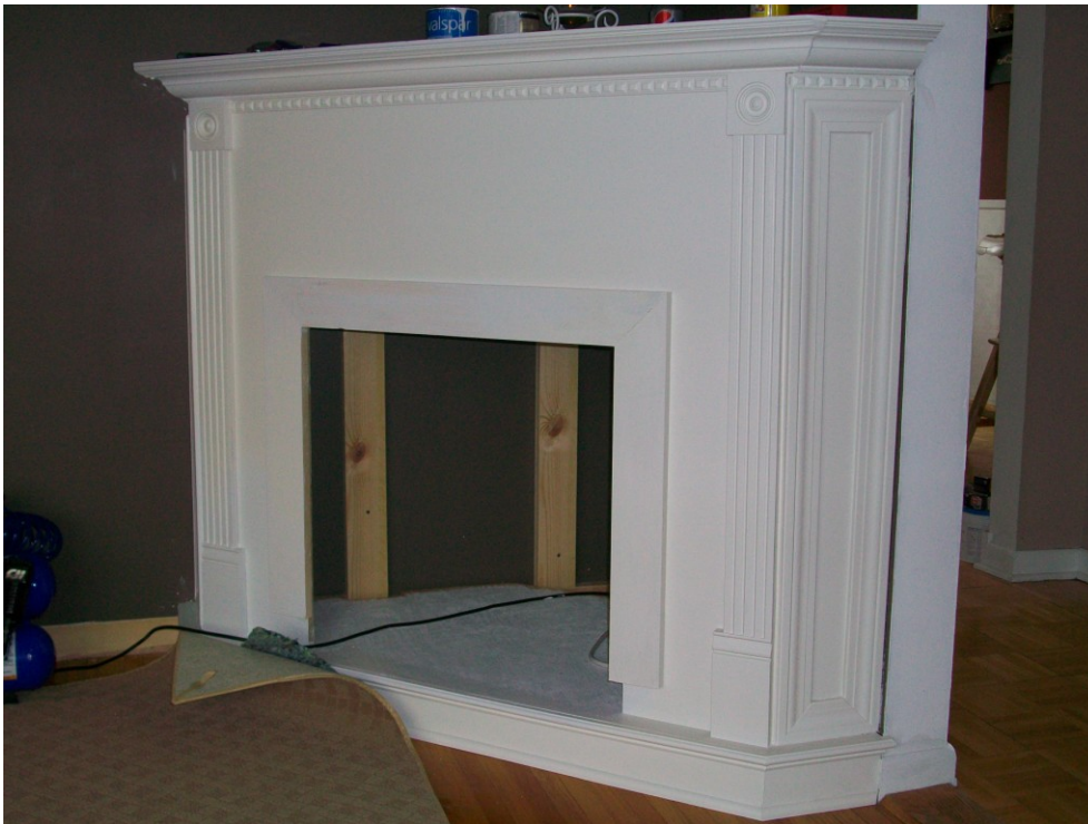
Figure B 24. Two coats of Valspar “Mystique” Interior Satin were applied as the finishing coats.
