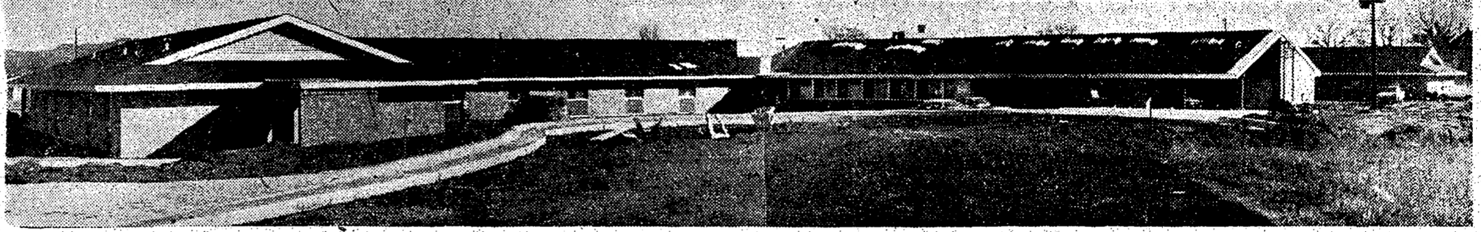
SAUER HOME . . . The three-quarter million dollar Sauer Memorial Home is now nearing completion at 1635 Service Dr. This view from the service entrance off West Mark Street shows at the extreme left the intensive care wing with a covered entrance. Adjacent to this in the center section is the administrative and service wing which will house administrative offices, dining-chapel and the dietary departments. The wing at the extreme right will house ambulatory and congregate care guests. The only basement is under the center section. In the basement are a barber-beauty shop, recreation room, physical therapy facilities, laundry, boiler room and storage facilities. The home will accommodate approximately 100 guests.
