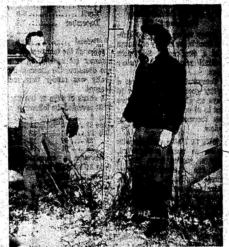
THE TOPPER... Winona's all-time record river stage of last spring was too high to be measured on the official river gauge at the Johnson Street pumping station so a new mark had to be written in above the top of the gauge which measures up to 20.30 feet. Shown are Donald Brown, left, and John Shugart, employees of the Board of Municipal Works, the latter pointing to the previous record high of 17.94 feet recorded in 1952. This year's new record crest of 20.75 feet was reached on April 19. (Sunday News photo)
