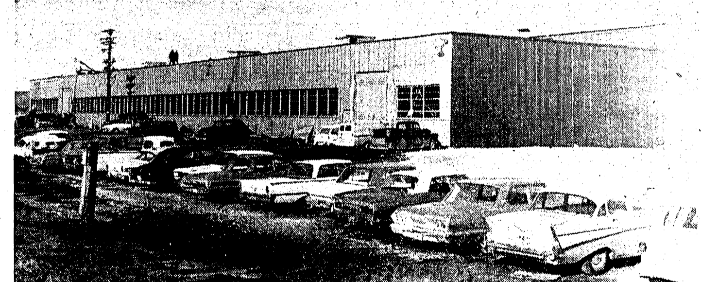
GROWING BIGGER . . . Warner & Swasey Co. continued to expand its Badger Division operation here with the construction of this 360-by-80-foot addition to its plant at 217 Airport Rd. in the Airport
