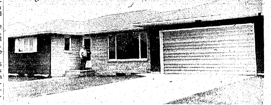
STONE ACCENT . . . A permit for construction of this house at 316 Emherst St., was drawn late last year by Hilke Homes, Inc., and is now owned and occupied by the Charles Stahl family. The house is 34 by 60 feet with attached garage and estimated cost of construction was listed at $13,000. (Sunday News photo)
