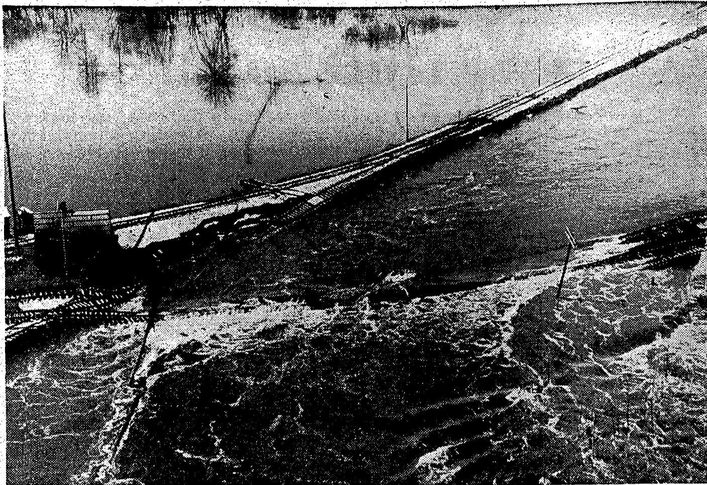
THE BREAKTHROUGH . . . Straining flood waters swirled through railroad right of way across the Mississippi River near Bluff Siding and Marshland, Wis., spilling into the lowlands. The opening momentarily eased the pressure on Winona's primary dike
