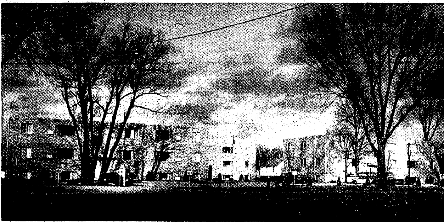
EAST SARNIA APARTMENTS . . . A major addition to the city's residential scene during the past year was the completion of this apartment complex on East Sarnia Street, on which work was begun last year. Each of the three three-story apartment struc-
