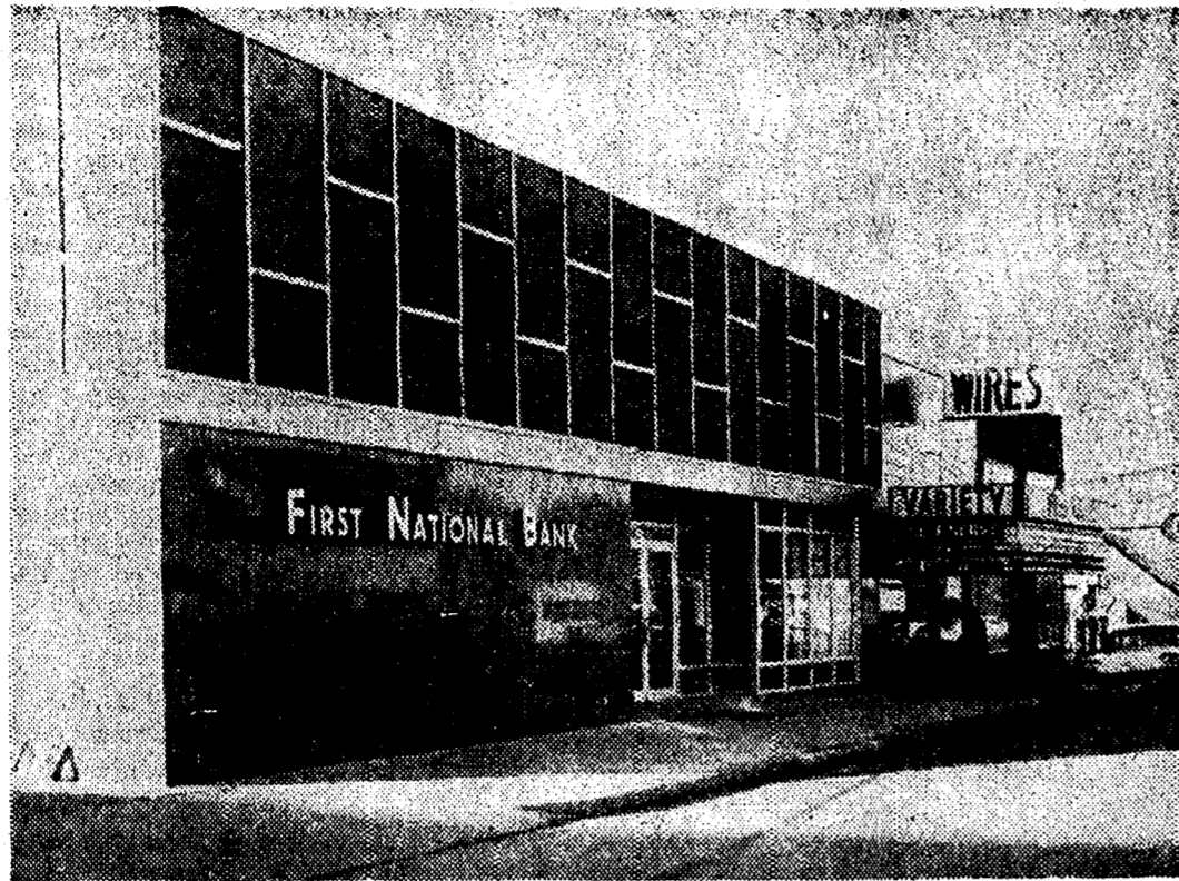
SPARKLING AND NEW . . . First National Bank in St. Charles is faced with red granite at the left and glass at the right of the Whitewater Avenue entrance. The material above is handsome anodized aluminum, painted gold. (Sunday News photos)
