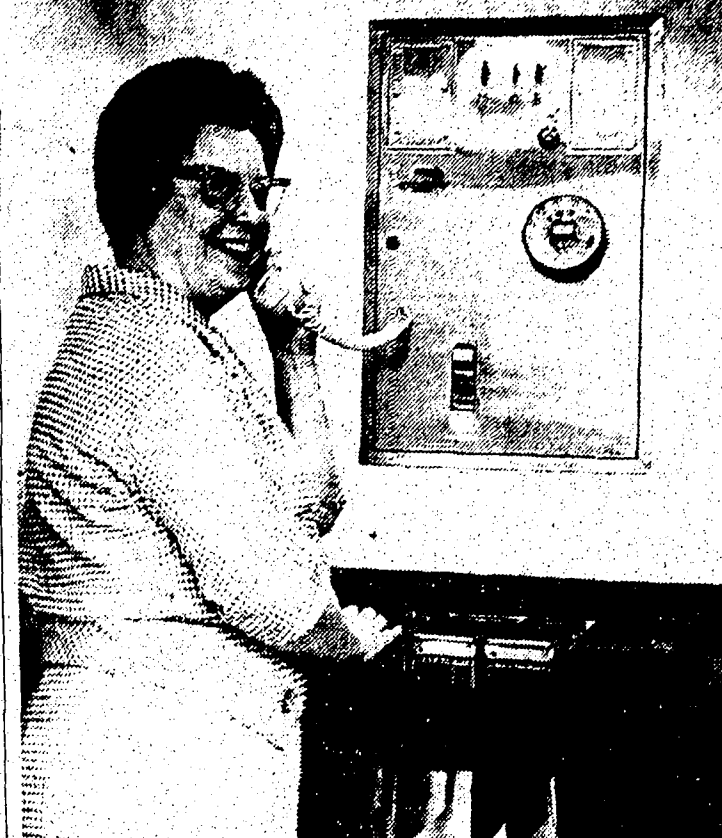
NEW PHONE BOOTH . . . Just inside the first door of the new Northwestern Bell addition on 3rd Street is this public telephone booth. All the equipment is included in a panel, which is set flush with the wall. Trying it out is Mrs. Harry S. Johnson Jr., 1283 Randall St., a telephone company employe.
