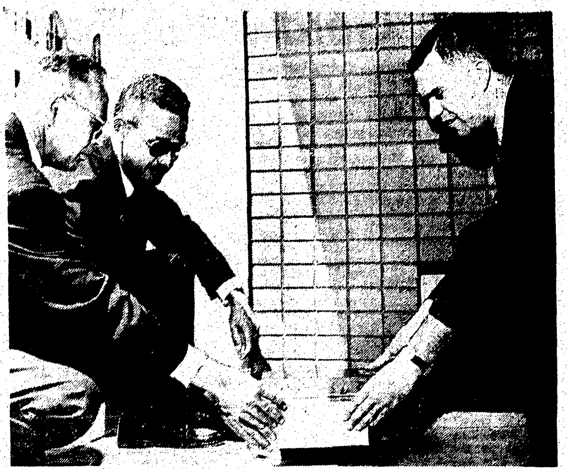
FOR THE FUTURE . . . Two of the guests at the dedication of the new Bell Telephone exchange addition help Robert C. Olson, the firm's manager here, put the metal box containing mementos of the ceremony into the cornerstone. From left are Harold Briesath, city council president; William Lang, Winona Chamber of Commerce president, and Olson. (Sunday News photos)
