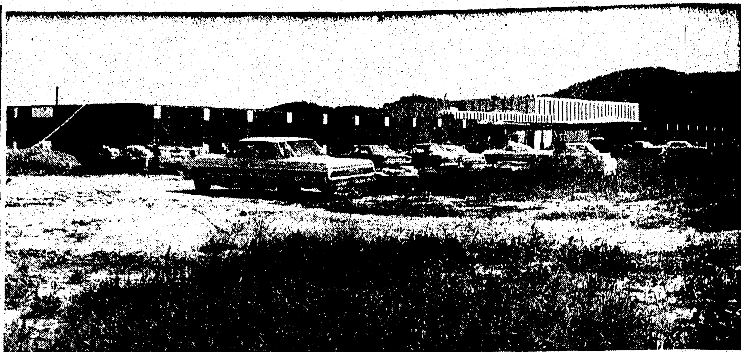
LA CRESCENT HIGH SCHOOL . . . Work is moving fast toward completion of the first high school at La Crescent, Minn., said Sidney Finley, Bloomington, supervisor on the job for George Madsen Construction Co., Minneapolis, general contractor. Interior work has progressed to the point of painting in some areas. The structure — for 540 students — will cost $1,153,741. The $1,400,000 bond issue voted by the village also will pay for furnishings. (Sunday News photo)
