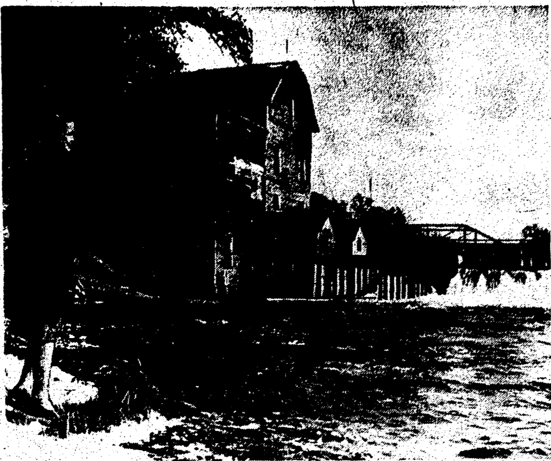
SAVED THE MILL . . . Miss Geneva Tweten looks over the old Phelps Mill site at Maine Township on the Otter Tail River near Fergus Falls, Minn., which she helped to save. Miss Tweten was instrumental in convincing the County Board of Commissioners to buy the site, which includes 18 acres. The flour mill, going back nearly 75 years, will be a historical and tourist site, if plans go through. (AP Photofax)
