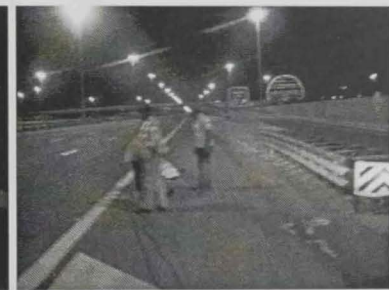
9. Installing the Pneumatic Tube
