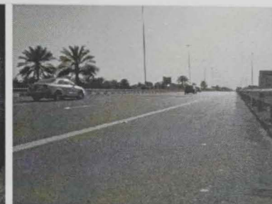
Pneumatic Tube on the road
