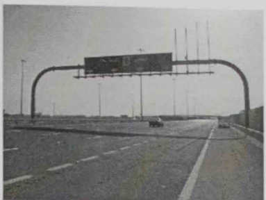
Pneumatic Tube on the road
