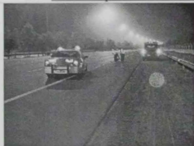
Team installing tubes
