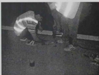
Team fixing the tubes on the road
