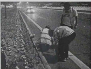
Team installing tubes with Police support
