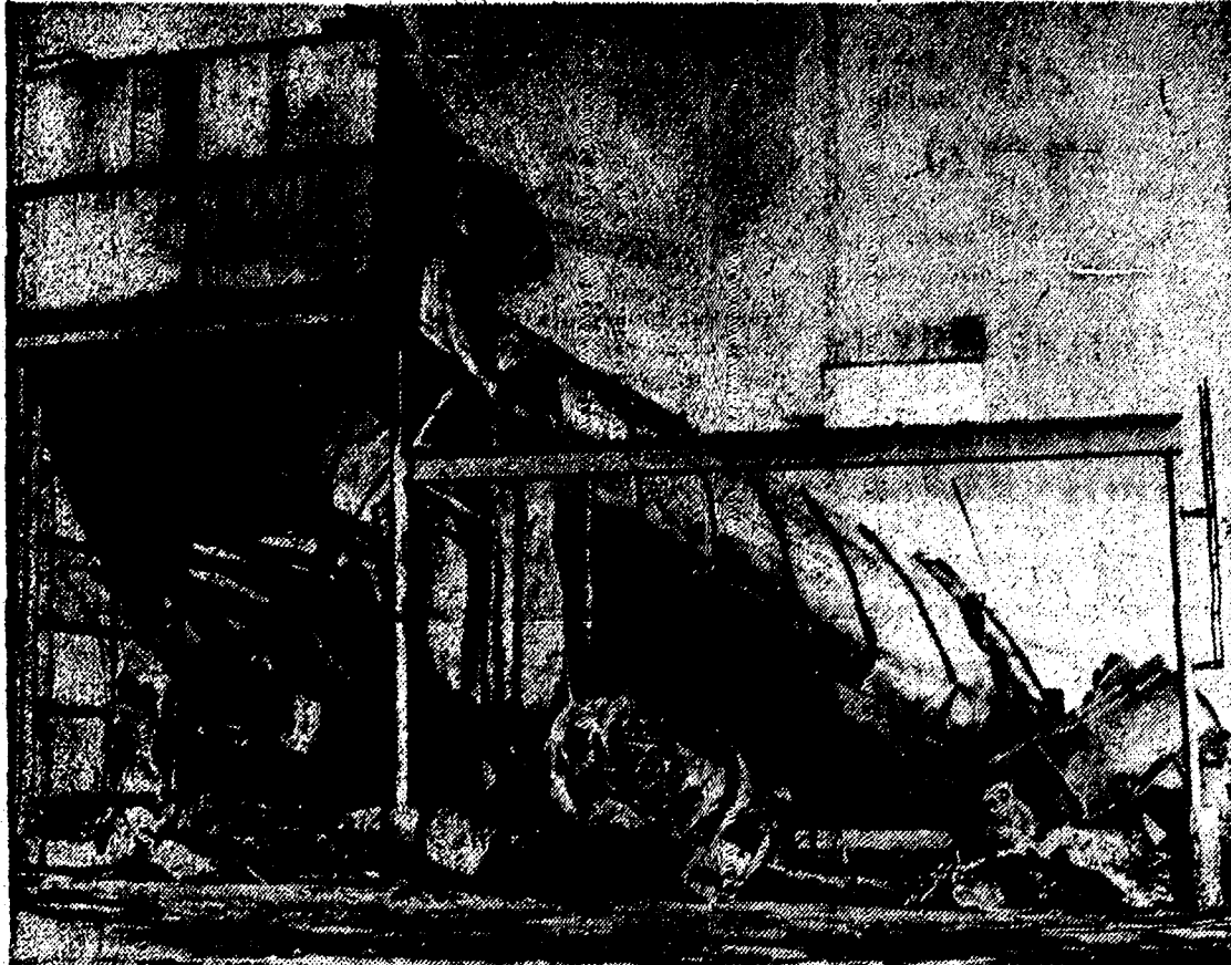
FEEDMILL HOLOCAUST . . . Fire Friday night destroyed a Mondovi Co-op Equity Association elevator and feed mill at an estimated loss of more than $200,000. Firemen from two departments fought the blaze in 10-degree temperatures. (Alton Nyseth photo)
