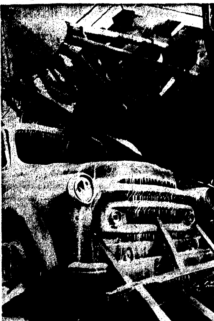
TRUCK LOST . . . Among the feed and equipment lost in the blaze was this truck which was coated with ice Saturday. Firemen were still pouring water into the smoldering structure late Saturday afternoon. (Sunday News photo)
