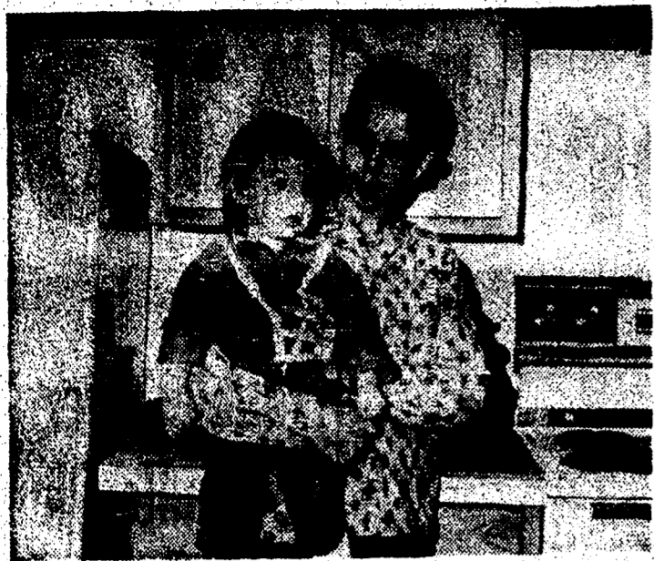
HOUSE THE KIDS BUILT . . . John Leisgang, 15, installed the kitchen cupboards, background, in the new Robert Leisgang home near Galesville. He's holding Pauline, 17 months, who picked up nails. All nine children in the family helped build the house. (Mrs. Dahlgren photos)
