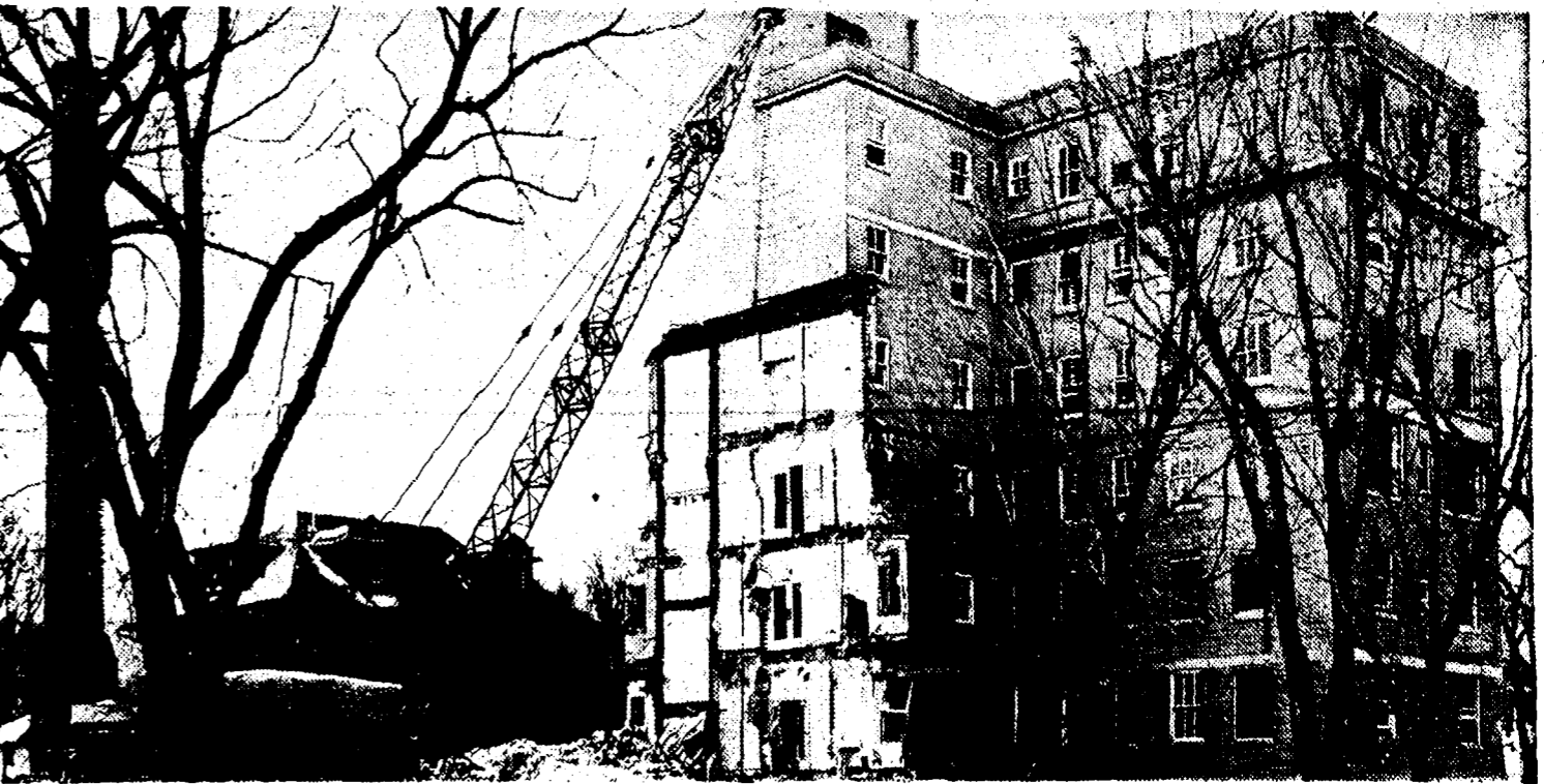
THREE FOR TWO . . . One of the city's landmarks, the old general hospital, gives way to wreckers to make room for a planned apartment development of three units. Razing of the building, vacant since last year, was started after hospital directors tried and rejected two other alternatives. They decided not to remodel it into a nursing home because of excessive costs and elected not to sell it because purchase bids were considered too low.
