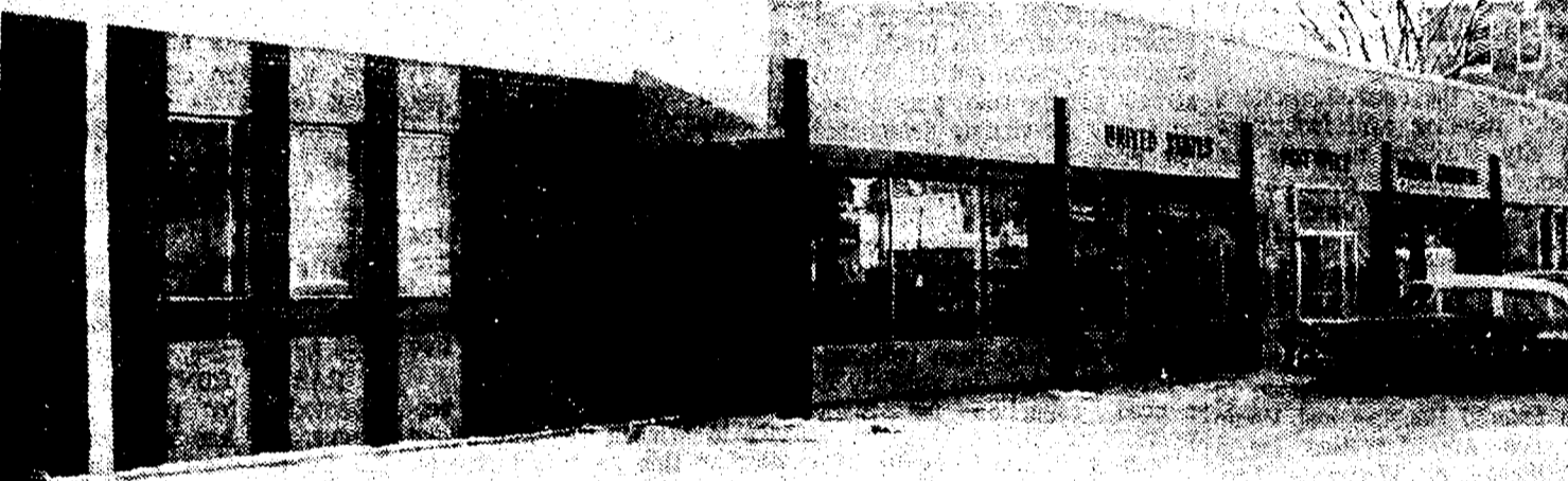
POST OFFICE COMPLETED . . . Construction of the new U. S. Post Office in Winona was completed early this year and now is in use. The permit for the $180,000 brick building, which faces West 5th Street and is between Center and Main streets, was
