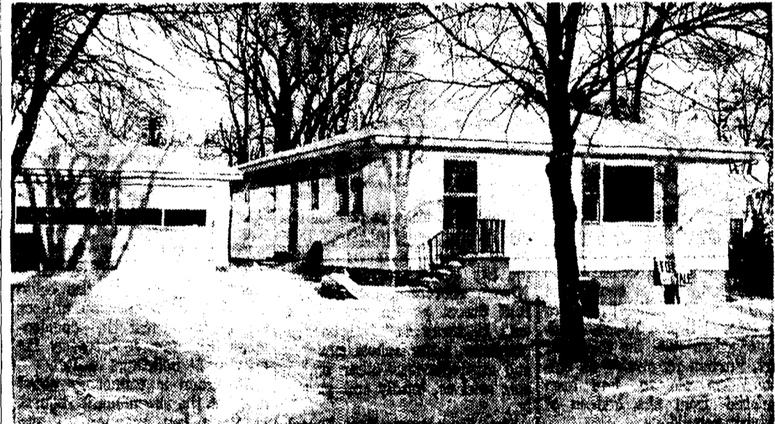
STUCCO FRAME HOME . . . Arne Odegaard was contractor for this 48-
