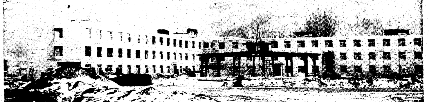
COLLEGE BUILDING BOOM . . . Assisi Hall Juniorate, rising in St. Michael's Field on the College of Saint Teresa campus, typifies the surge in college construction that boosted Winona's employment rate to record levels during 1963. In addition
