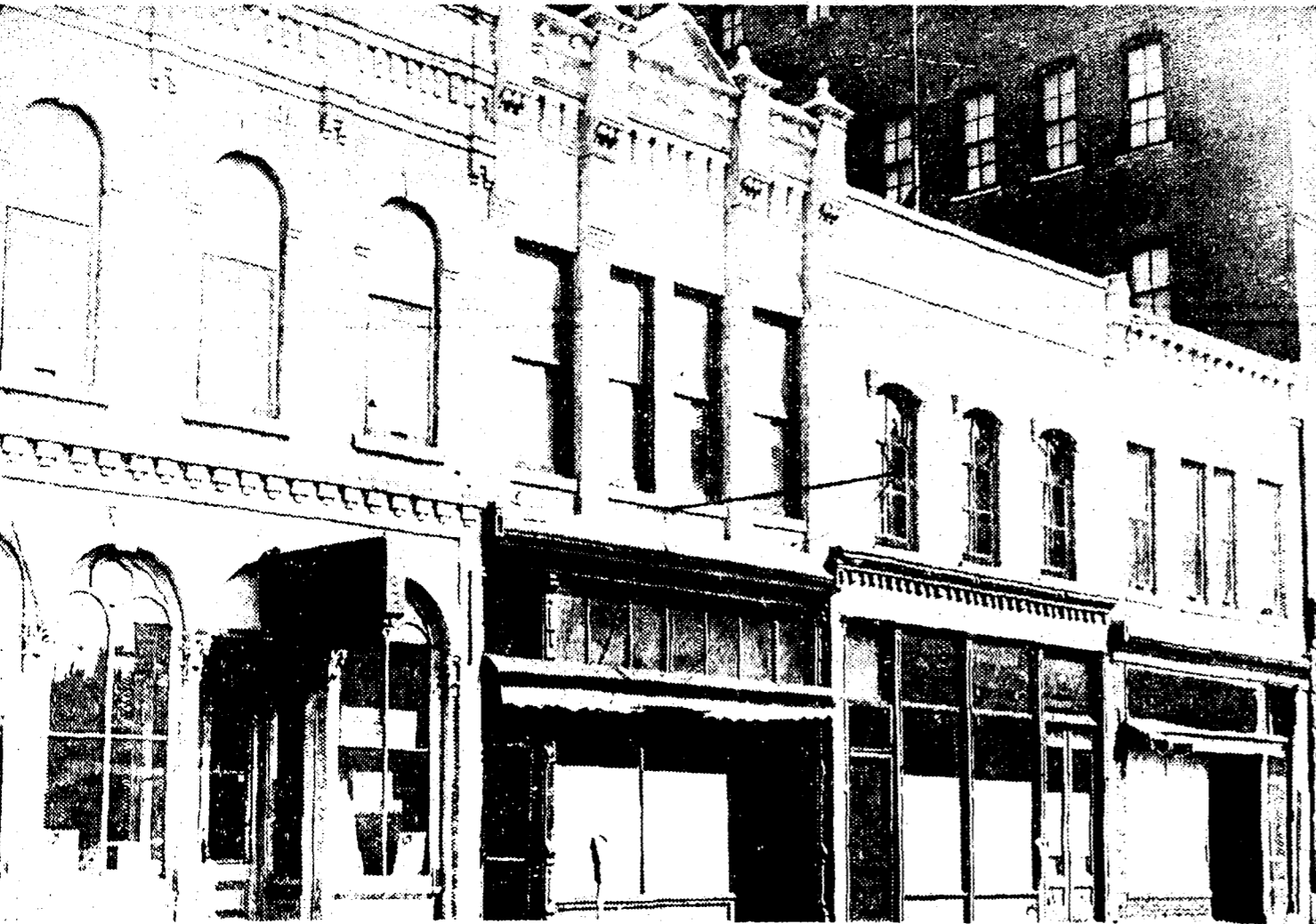
UPDATING: WHERE OR WHEN? . . . Old buildings, a bountiful commodity, were more than ever in the limelight this year as steam built up under the urge for downtown redevelopment. Opposition was voiced against the "bulldozer approach" and against the pursuit of federal grants to help finance the
