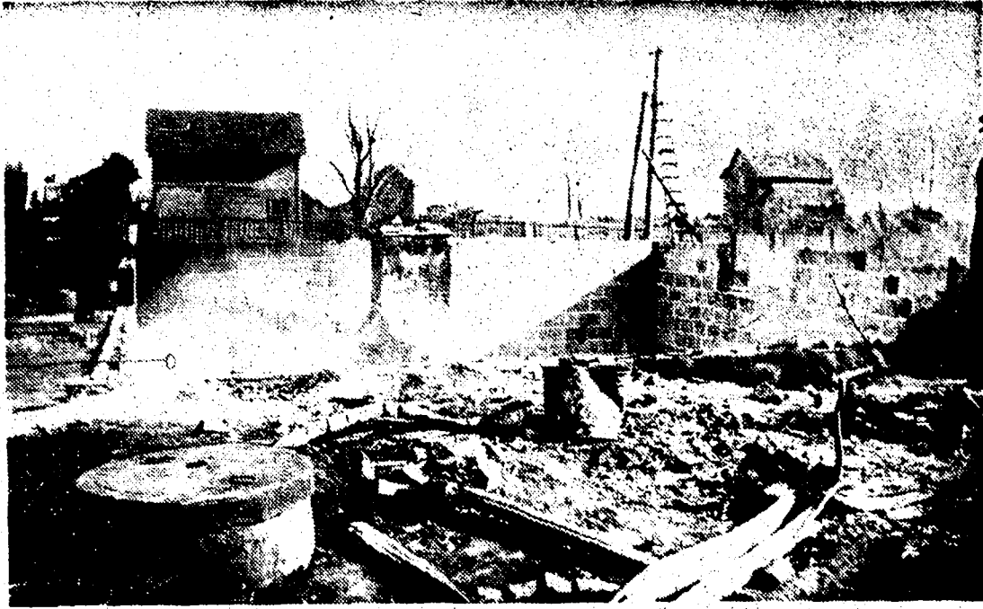
THE FLAMES LEAPED... This is all that remained of the Frank Frye residence after a disastrous early morning fire that destroyed four buildings in Hesper 40 years ago.
