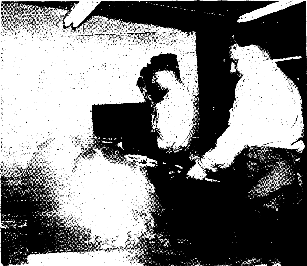
NEW FINISH . . . Each article reaching the tinning line has three baths in molten tin. Tony Pehler, left, and Edgar Feine here are immersing 20-quart mixing bowls in the tin baths.
