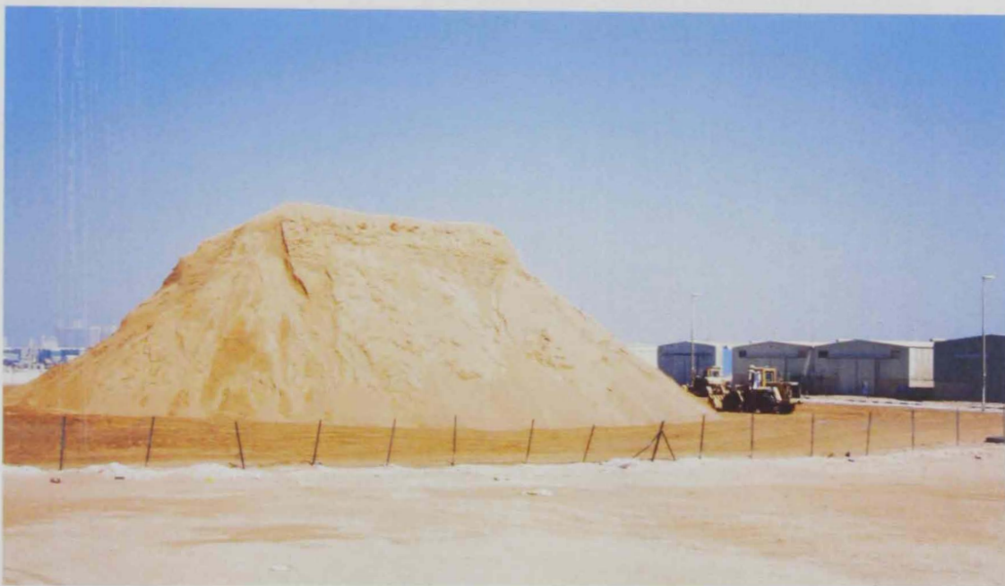
Figure 4-29: Huge amount of earth have been moved and transported to reclaim land from the sea in many parts of Abu Dhabi coastal area. The photo is showing an example of a huge pile of earth which is ready to use for reclamation purposes.
