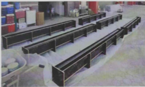
(a) Fabricated formworks
