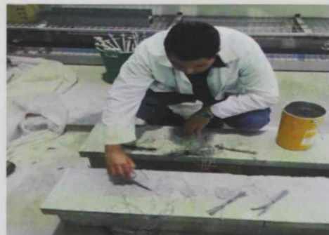
(d) Removal of extra epoxy and finishing of concrete surface.
