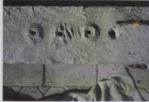
(b) Holes after drilling
