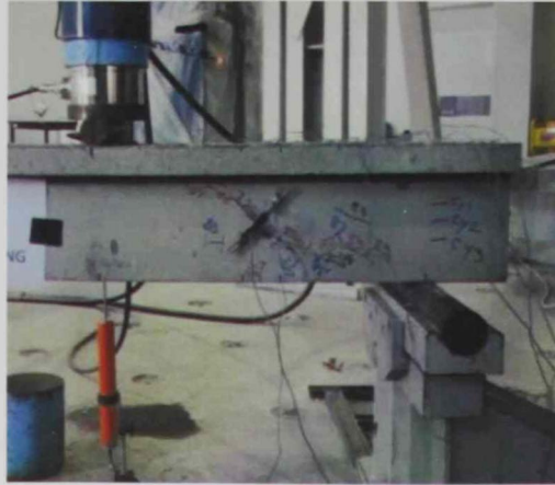
After initial shear damage D1
