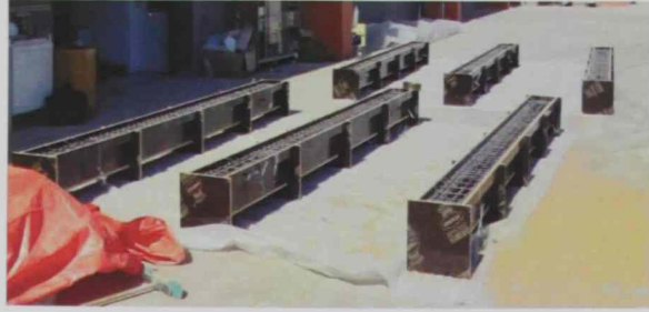
Figure 3.8: Installation of steel cages in the forms before casting
