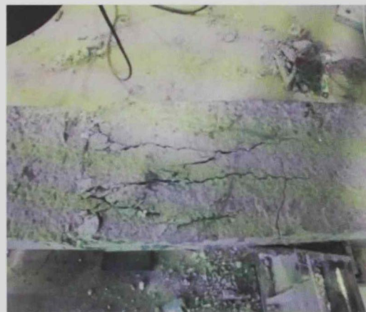
At failure (Top view)
