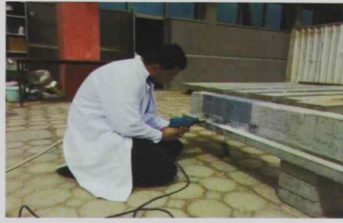
(b) Drilling of holes for the anchor bolts
