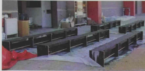
Figure 3.9: Concrete after casting
