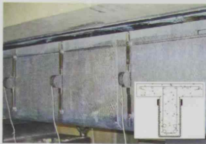
SBFA anchorage system
