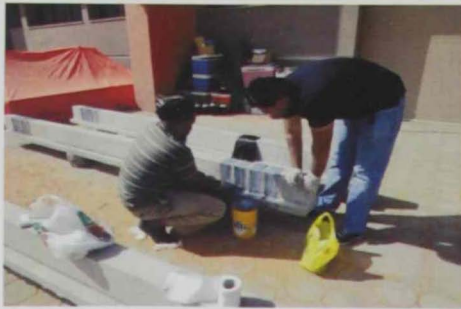
(c) Application of the final sealer coat
