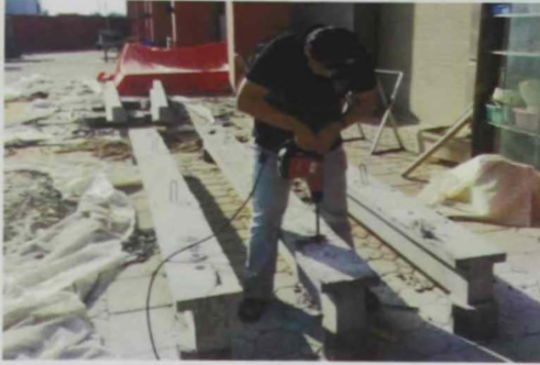
(a) Drilling of holes through the beam depth
