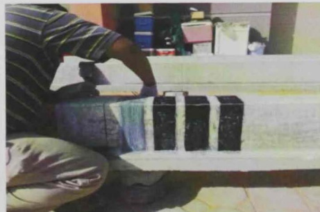
(b) Bonding of the CFRP sheets to the concrete
