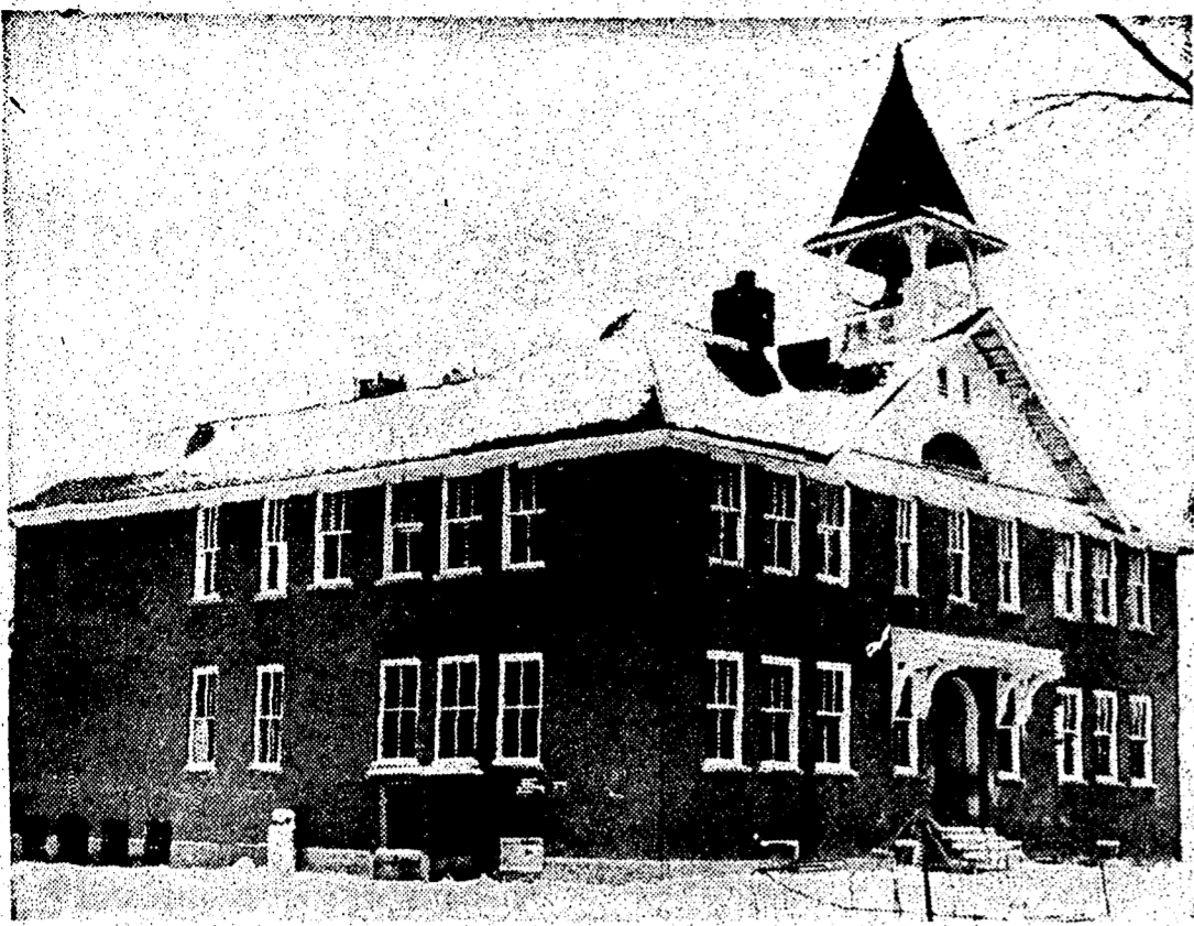
TO BE DEMOLISHED . . . Bids will be received by Independent School District 811 in the board room at Wabasha Public School Feb. 6 for the sale for demolition of this old school building at Kellogg. The building and walls must be reduced to one foot below ground level by Sept. 1. All debris must be removed from the site except sufficient masonry debris to fill the basement to one foot below ground level. All other salvage material will be the property of the contractor. Bids will be opened at 8:30 p.m.
