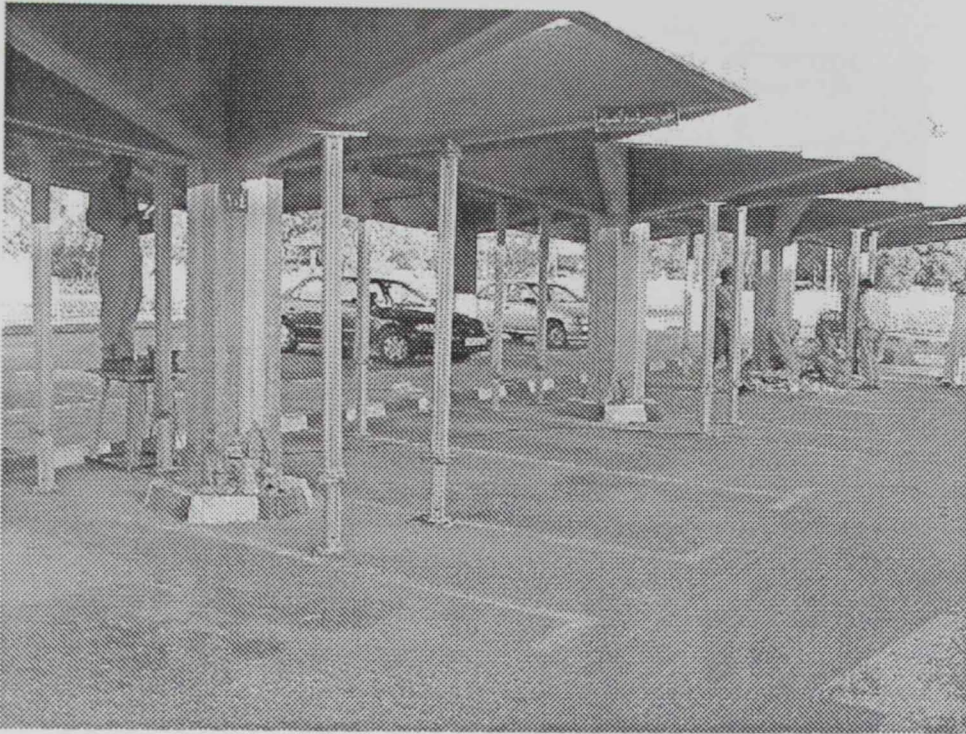
Figure 3-7 the columns were chosen for testing
