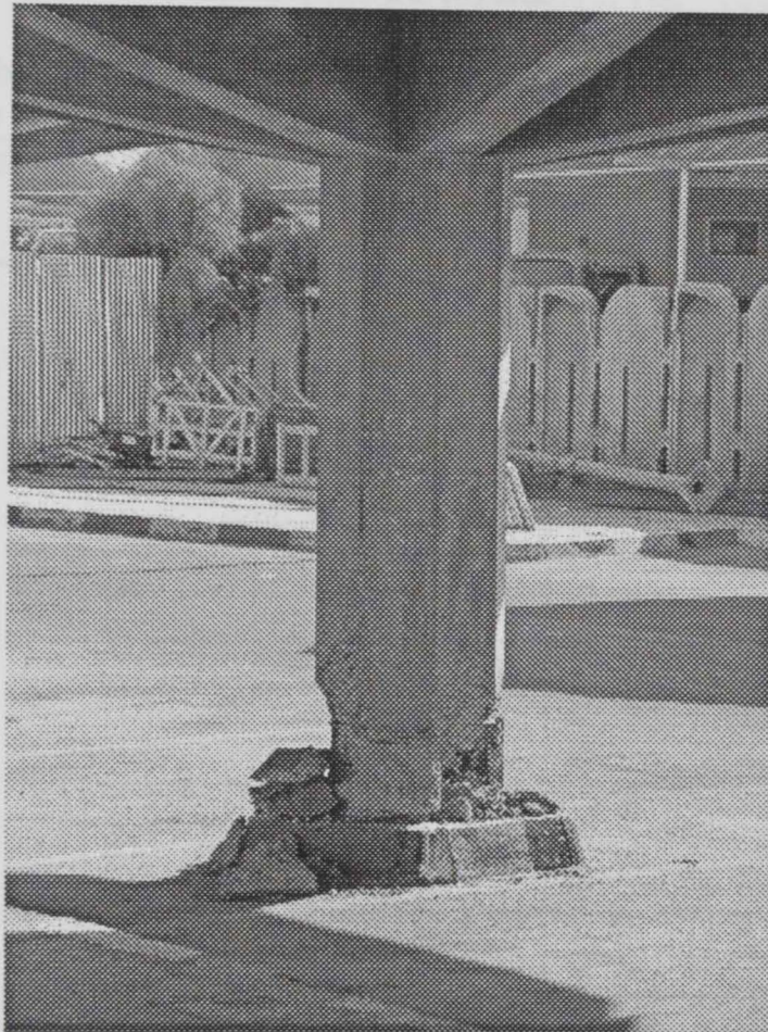
Figure 3-4 Initial state of column C1 before repair
