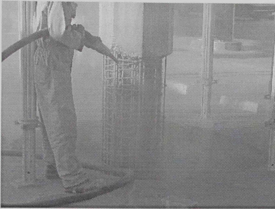
Figure 3-9 Concrete sandblasting with shotcreting equipment
