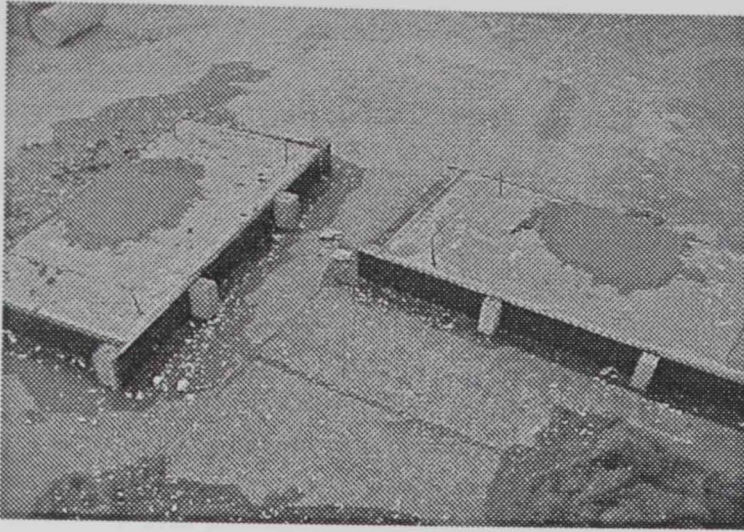
Figure 3-16 Location of large repaired area
