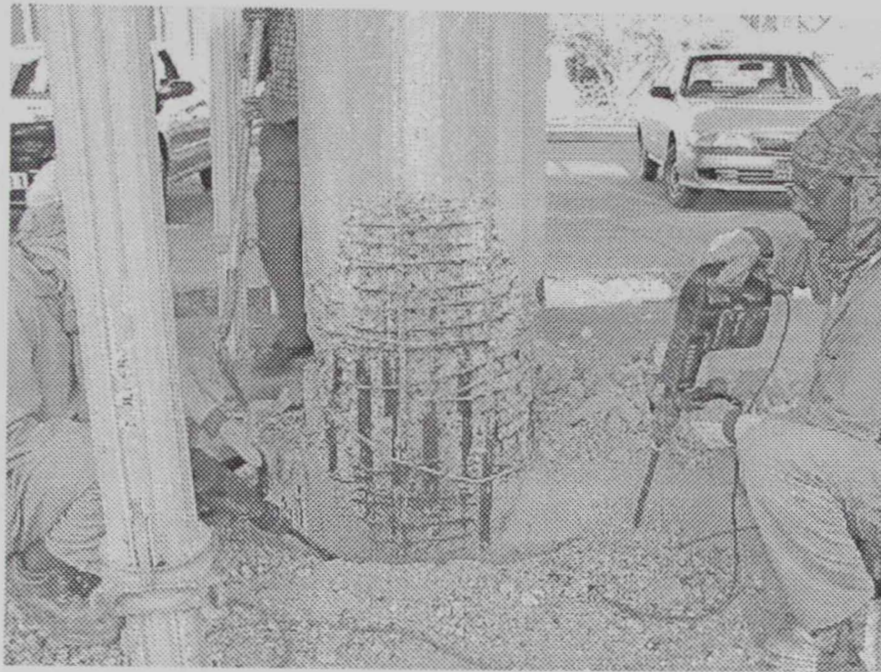
Figure 3-8 Breaking out deteriorated concrete using pneumatic hammer
