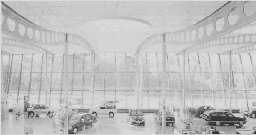
(b): Cellular Beams as Structurally Exposed Elements
