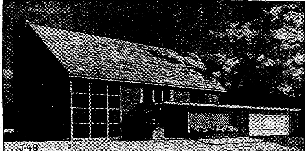
NEW CONCEPT: This house can be termed a "raised 1 1/2-story," since it combines a bi-level (with its mid-level entry and basement) with a story and a half (which has a steep roof pitch to make the attic habitable). The house contains five bedrooms plus all the other rooms a large family requires, yet covers only 930 square feet of ground area.
