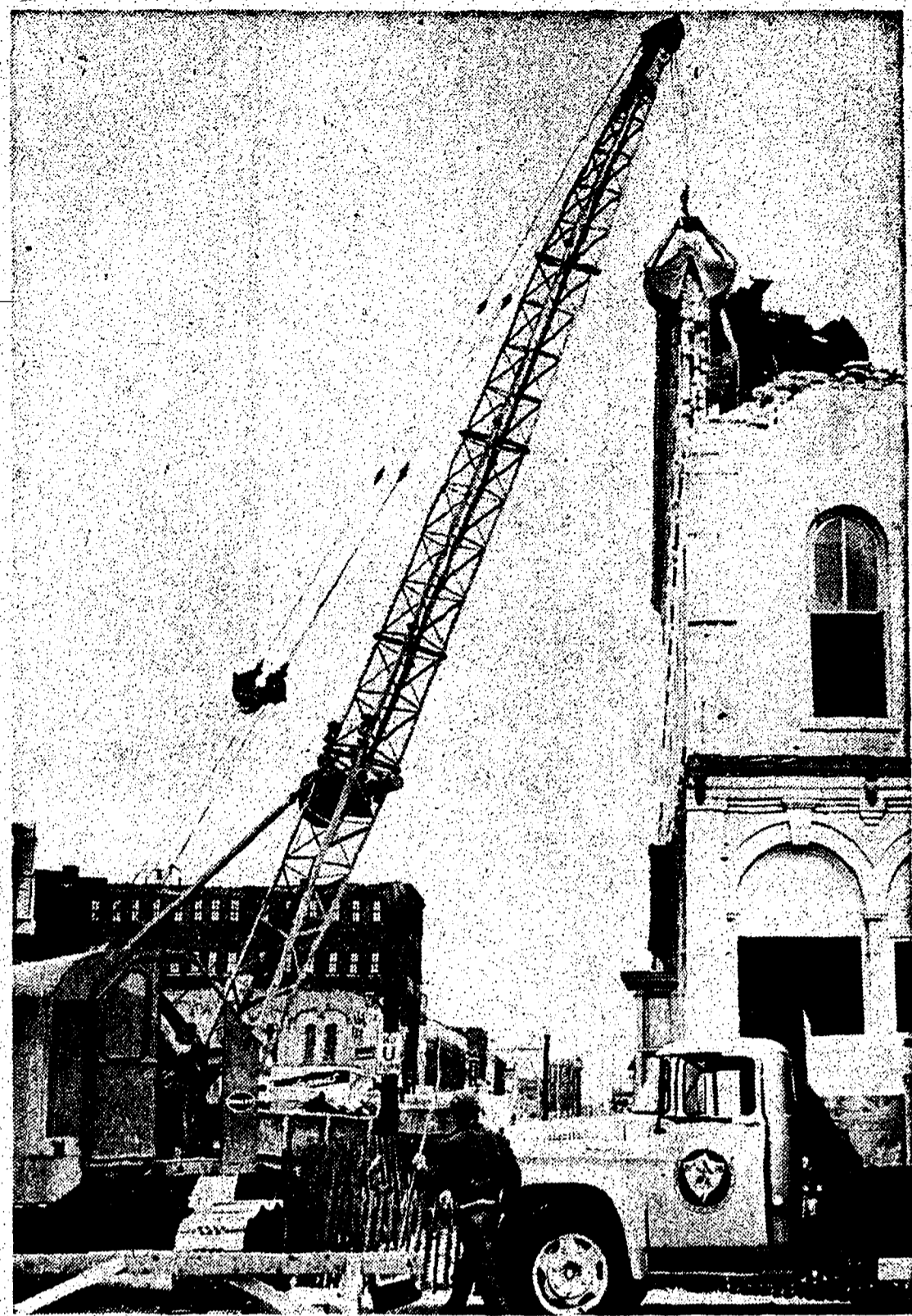
WALLS TUMBLE DOWN . . . Somewhat like a fictional monster, an excavating machine takes a bite of brick wall from the old Park Hotel building. Wrecking operations on the old landmark are expected to be completed within two weeks. Soon to rise on the site at Main and 2nd streets is the new A & P building. Some of the footings for the new supermarket will be poured next week. (Daily News photo)
