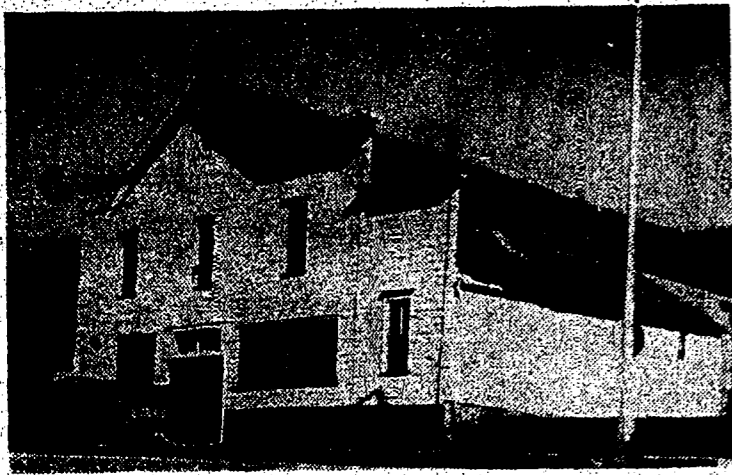
THEY HAVE TO GO... Progress has decreed that this large white building, used as a skating rink, and the building to the left must be razed to make room for a new post office under construction in Lanesboro. (Vienna Drake photo)
