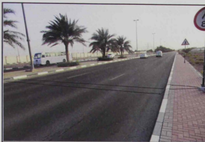
Figure 4.3: Khaled Bin Sultan Street Snapshot (Source: DOT)
