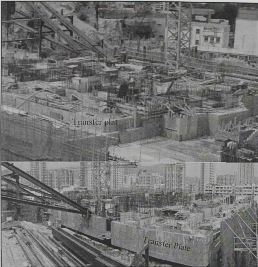
Figure A.11: Residential Development in To Kwa Wan - building 12 (Wong, 2013)
