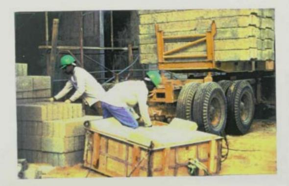
Figure (6): Unsafe Act (improper Lifting)
