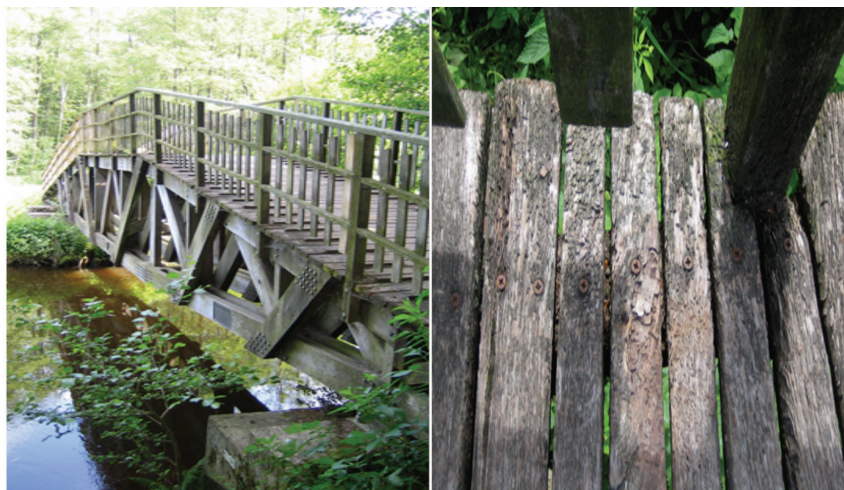
Figure 1. Investigated bridge and detail with fruiting bodies (Lerche 2010).
