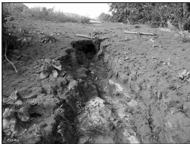
Obr. 4: Fotodokumentace výtoku č. 1 mezi patou haldy a cestou. Fig. 4: Photodocumentation of the outflow No. 1 between the base of the slag heap and the road.
