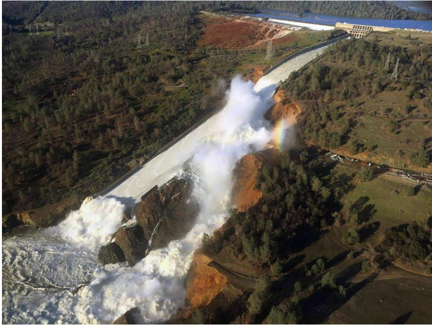
Record rains and flooding in N. California damaged the Oroville Dam.
