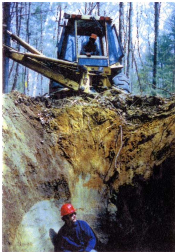
Figure 6.1 Trench was 3.2 m deep by about 35 m long. Cobble in foreground is 24 cm long.
