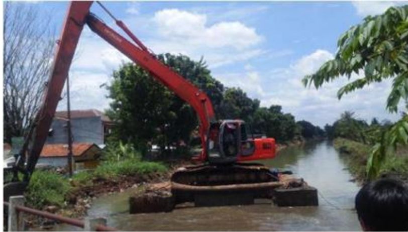
Figure 3. Dredging of Kali Baru river (Author Documentation, 2016)
