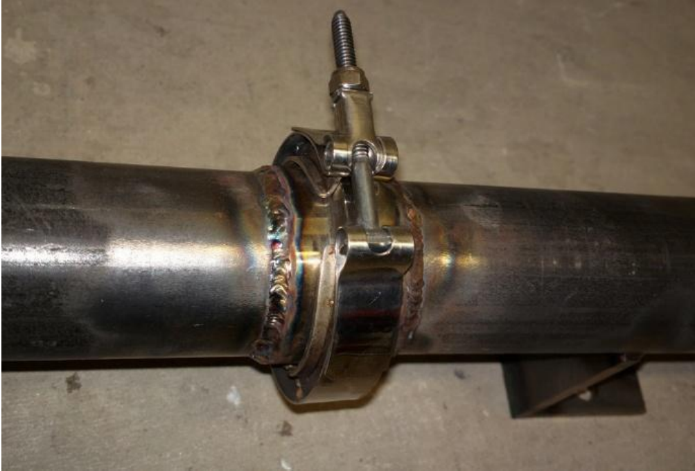
Figure 13: Previous two sections joined and clamped together.
