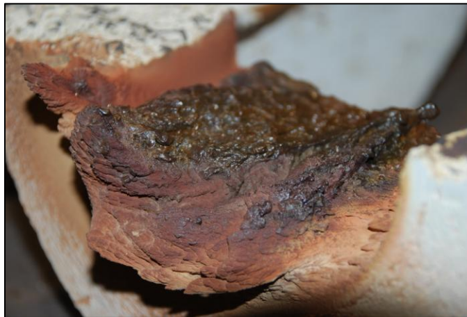
Figure 5.23. Image of deposit structure on transition piece after removal from aerothermal test section.
