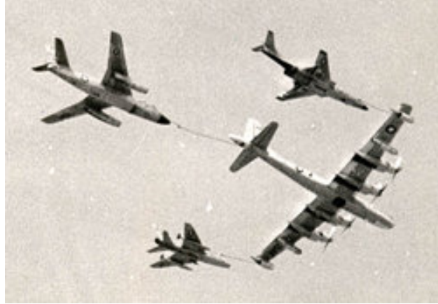
Figure 1.1: An early 1960's aerial refueling technique
