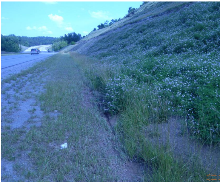
Photo 2: Limited distance between roadway shoulder and toe of slope.
