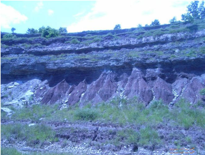
Photo 2: Mounds of erosion from highly friable Redbed shales at Location 4.
