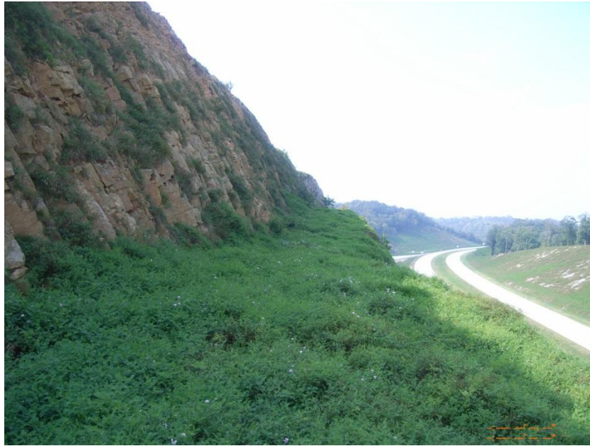
Figure 6.2 Vegetative cover on bench and portions of backslope on the US Rt. 48 Cut Slope Section
