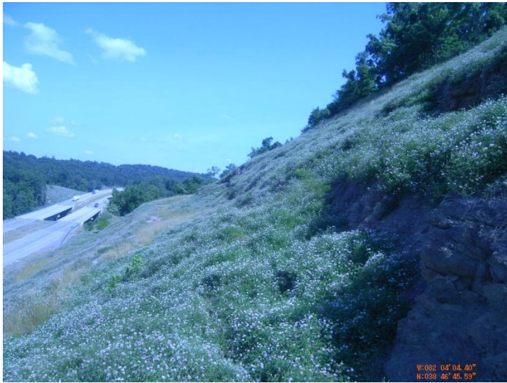
Photo 1: All backslopes and benches highly vegetated.
