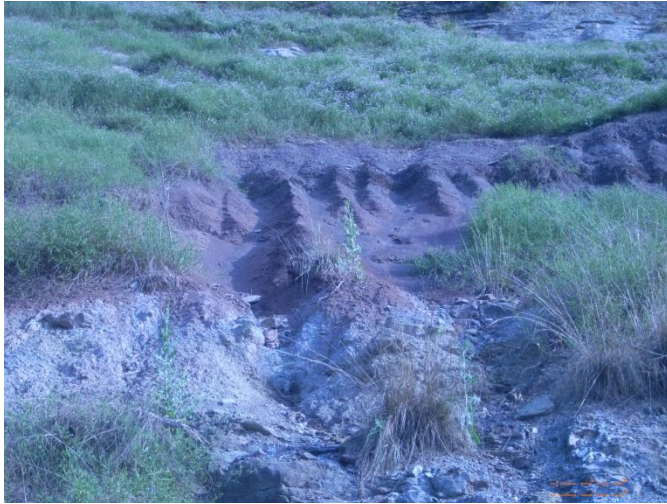
Photo 1: Rills and gullies formed on lower backslopes.
