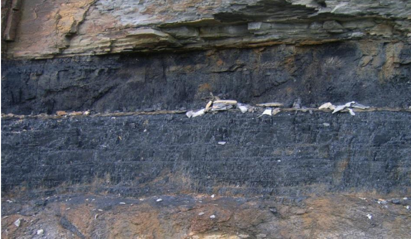
Photo 1: Large undercut above a coal seam at Location 2.
