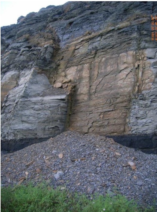
Photo 2: Extensive eroding of siltstone layers on lower benches at Location 2.
