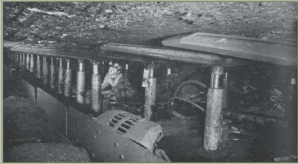
Figure 1-2: Longwall Face at Sunnyside Mine Using Self-advancing Hydraulic Roof Supports ("Frames") 2
