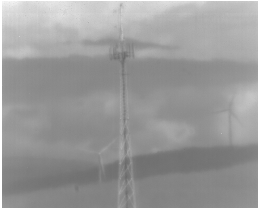
Figure 48 Radio Tower and Wind Turbines
