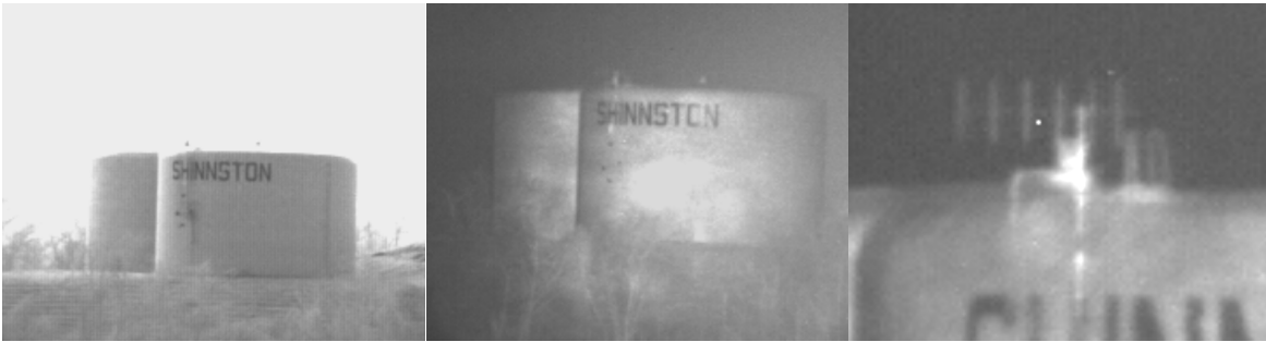
Figure 47 Shinnston Water Tower
