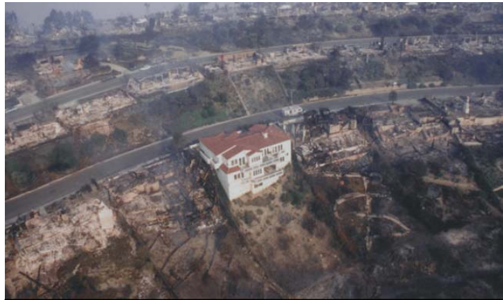
Figure 8-52. Fire resistance capability of aerated concrete block is shown by this house which survived devastating fire in California.
