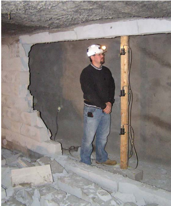
Figure 4-14. Photo after the wall was destroyed from the transverse loading. Researcher is standing next to the displacement transducers used to measure the wall deflection.
