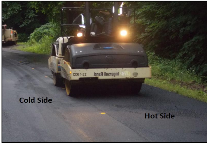
Good roller placement hot-to-cold (Project Id 66)
