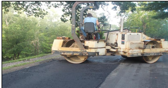
Good Compaction perpendicular to paving direction (Project Id 80)
