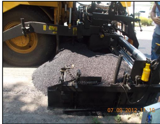
Poor (Project Id 70)
