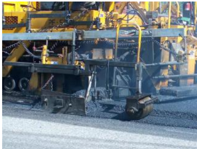
Figure 2-29 Wedge Joint (Pavement Interactive)
