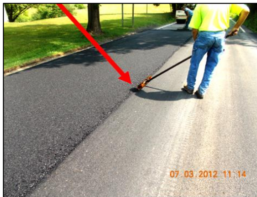
Good longitudinal joint luting practice (Project Id 68)
