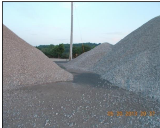
Fair base condition (Project 142)
