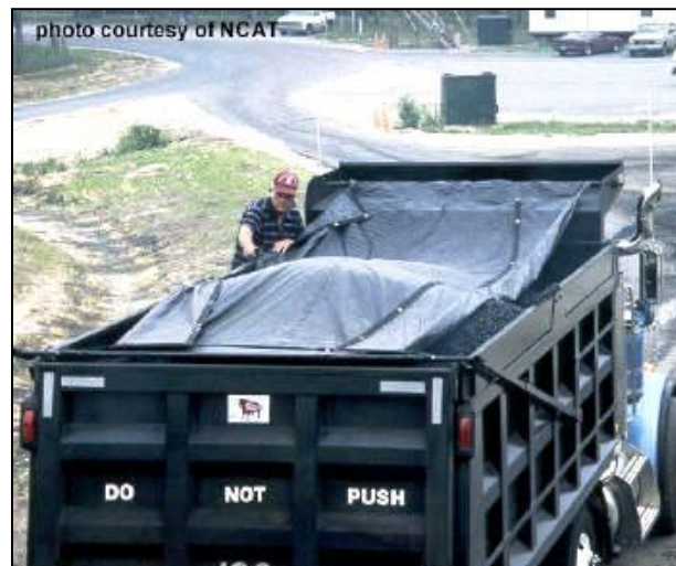
Figure 2-20 Tarp provides less heat loss (Pavement Interactive, 2014)
