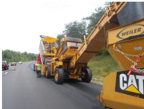
Figure 2-22 Material Transfer Vehicle without Remixing
