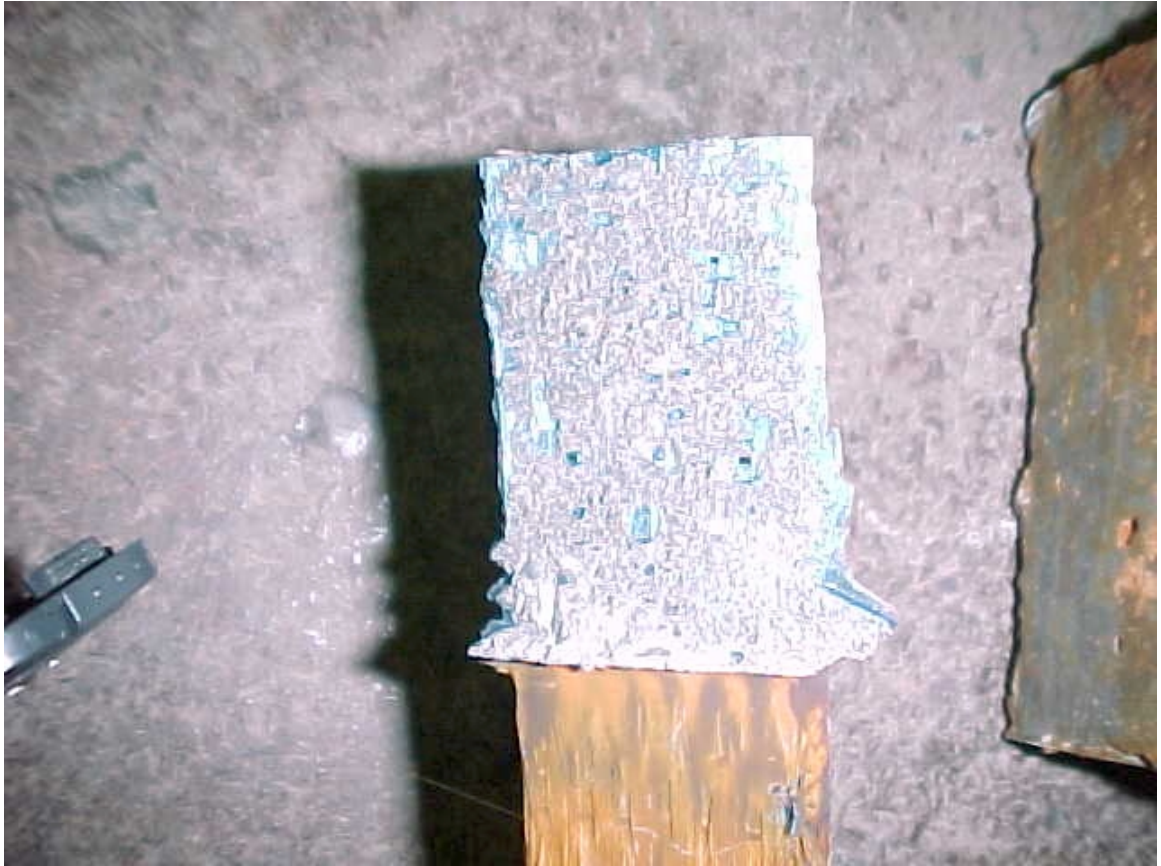
Figure 5.38 Thin Layer of Concrete Remaining on Strip
