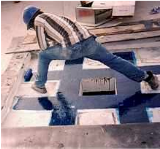
MBrace used to reinforce new slab opening
