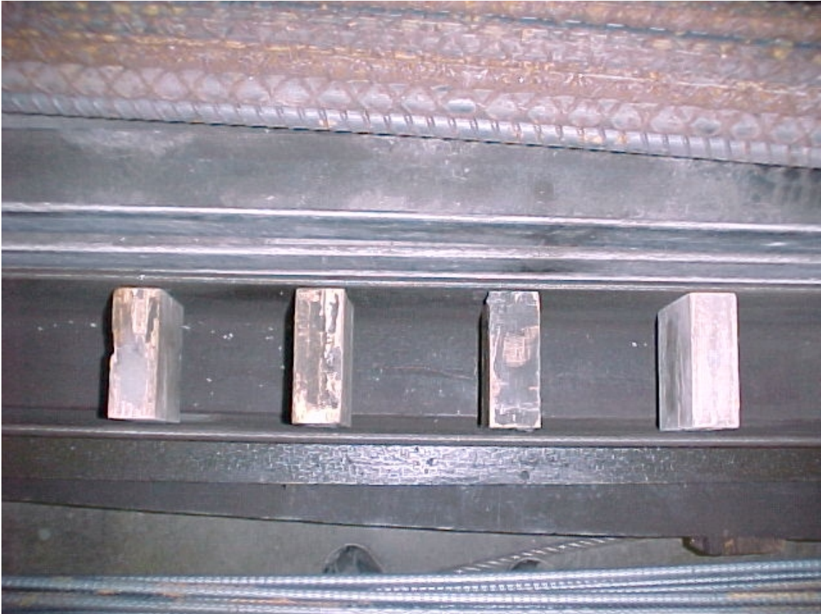
Figure 4.1 Formwork for concrete cubes
