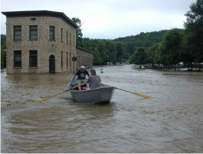
Figure 2: Flood waters inundated the former bank of Glen Jean, which is listed on the National Register of Historic Places (National Park Service photo, 2001).
