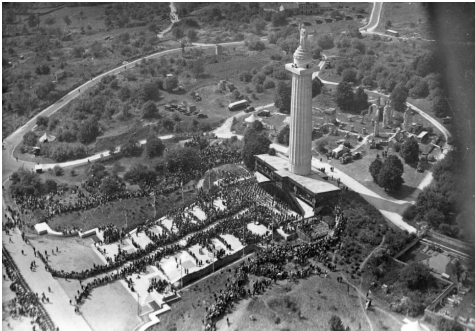
Photo 3.6.: Aerial view of Montfaucon Dedication, August 1, 1937. Source: ABMC Archives, Arlington, VA.
