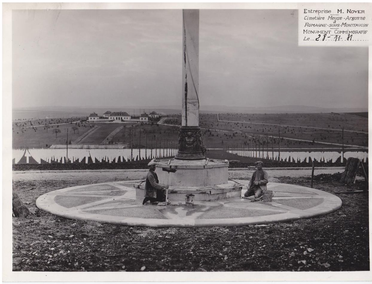
Photo 3.1: French Laborers completing masonry work on Meuse Argonne American Cemetery flagpole, November 1928. Source: RG 117 National Archives.
