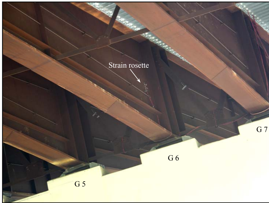
Figure 4.10 Shear Rosette at its Final Stage
