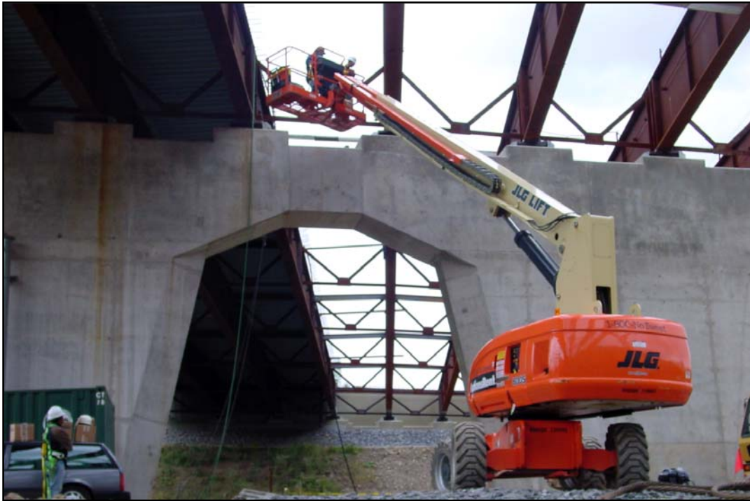
Figure 4.27 Accessibility of Sensor Location by use of Man-lift
