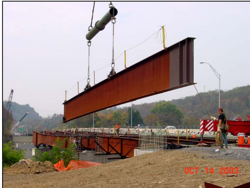
Figure 3.7 Erection Operations of Steel Girders.
