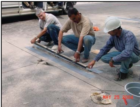
Placement of Peizo-electric sensors
